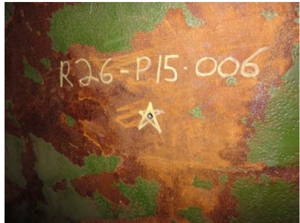
Port 006- R26 Plate 15; Drilled
