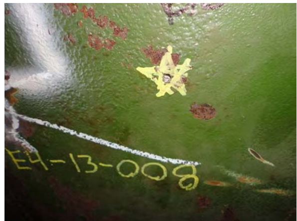
Port 008- E4 Plate 13; Drilled
