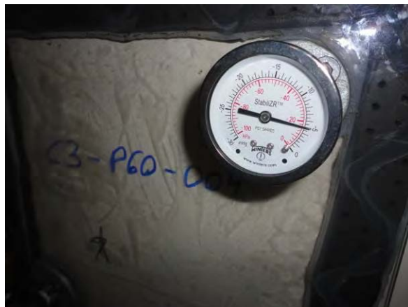
Port 004- C3 Plate 60; Vacuumed
