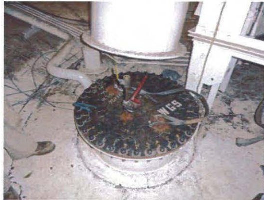
Figure 11.0: The custom fabricated 32"Ø ported flange supplied by WGS is shown here.
