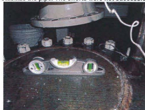
Figure 7.0: As we exhausted methods to rule out trapped air in the 18"Ø line, we decided to see if the level of the flange inside of the tank could trap a small amount of air and the conclusion is yes. (See drawing 6-1)
