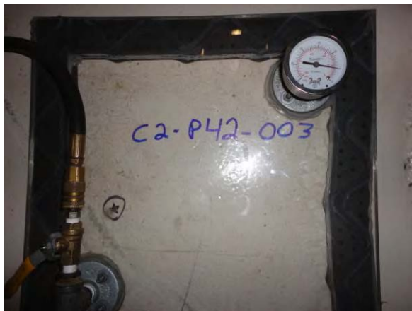
Port 003- C2 Plate 42; Vacuumed
