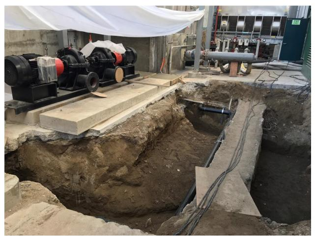
A picture containing a large excavation site where underground piping was replaced.
