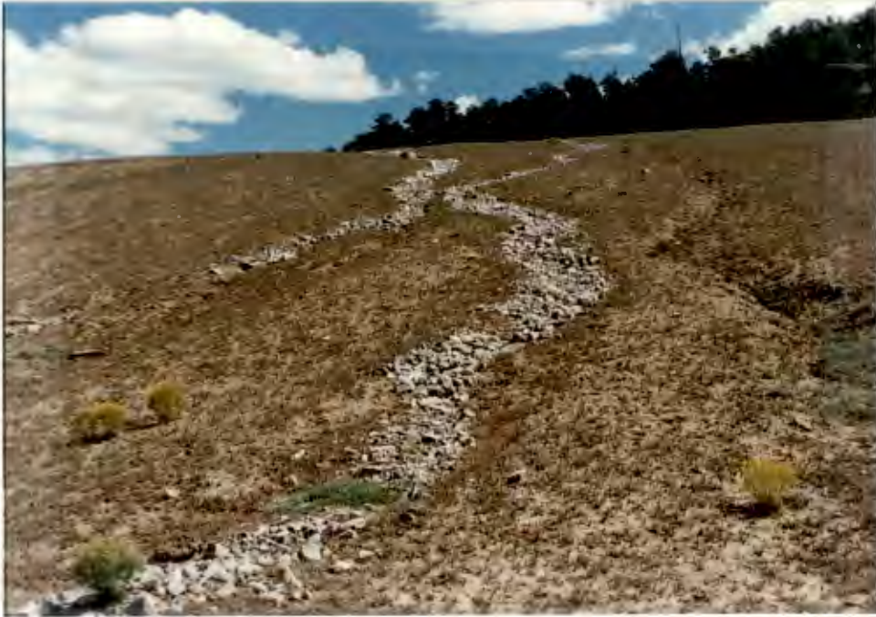
Ruby 1 Mine Repaired Erosion Features
