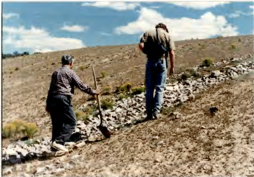
Ruby 1 Mine Repaired Erosion Features
