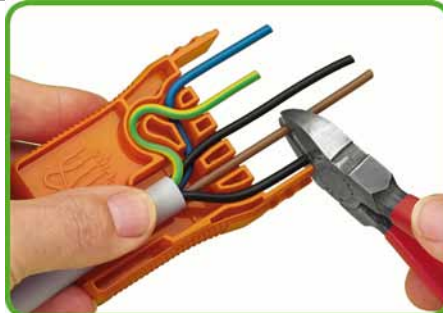
Cut conductor ends.
