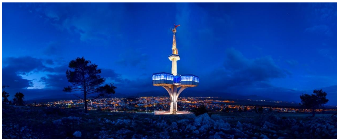
Main control-measuring center on Dajbabska gora in Podgorica
