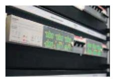
Measurement slot-in unit with extensive measurement functions (local or remote) Can be integrated into various management programs.
