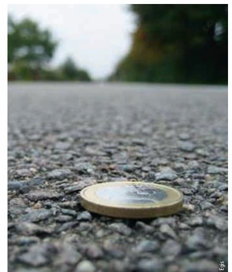
Photo 10 Aspect final de surface de la couche de roulement Final appearance of wearing course
