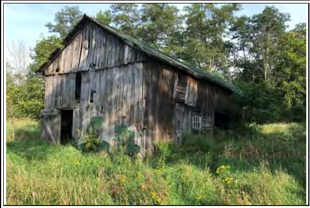
Photo 3 – Exterior of old barn in northern area of site
