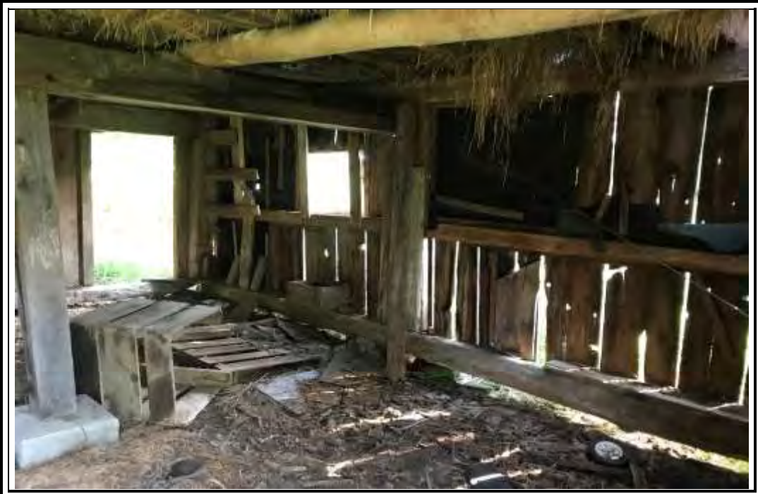
Photo 4 – Typical of interior of barn
