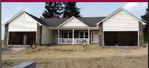
11 Par Lane $169,900 Experience the newest in one-level, maintenance-free living in The Meadows. Enjoy the beautiful Golf Course views of Meadow Ponds. Walk the cart paths in the evenings. Three bedrooms, 2 bathrooms and 2-car garage. 1316 square feet finished open floor plan.
