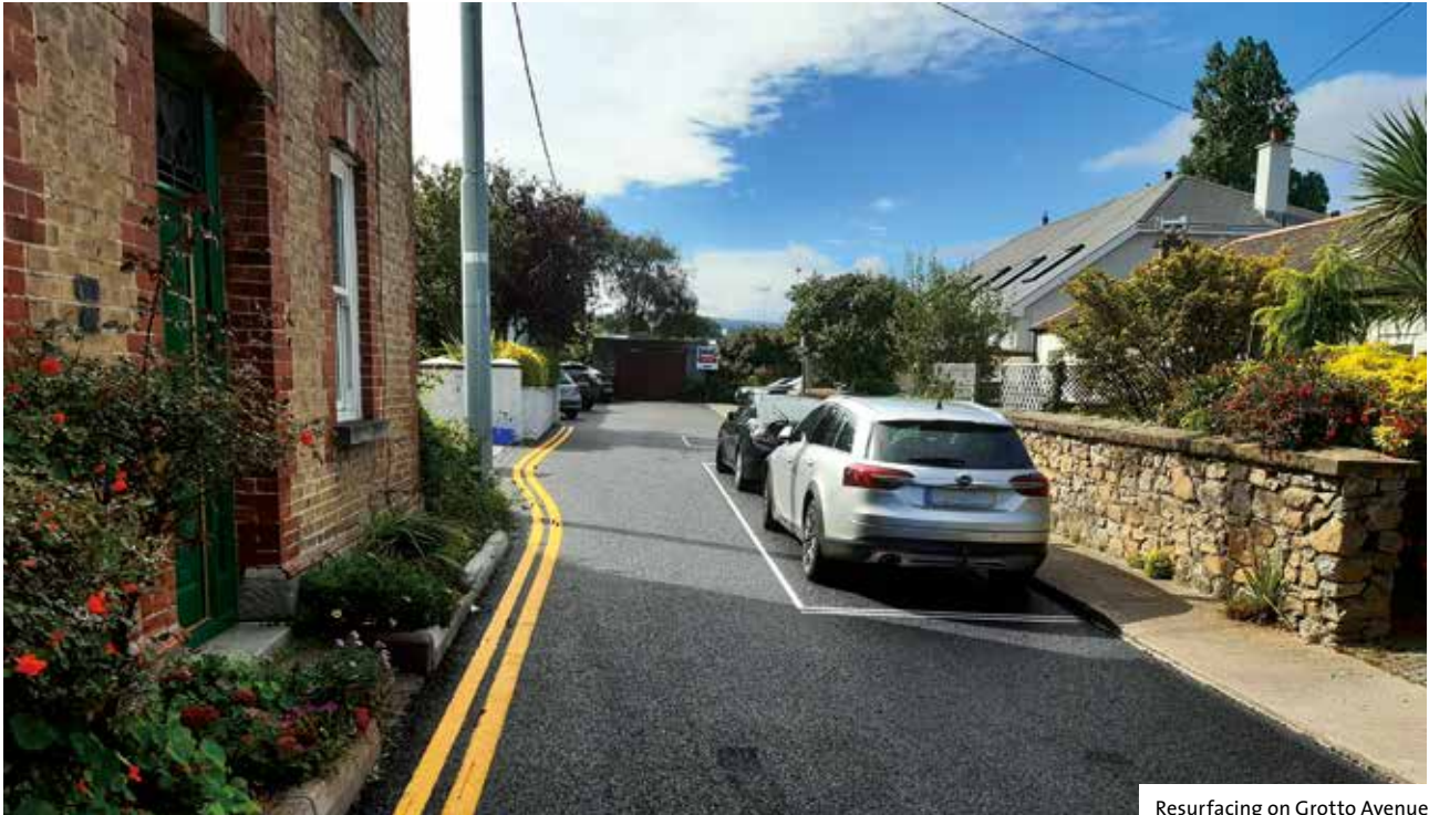
Resurfacing on Grotto Avenue
