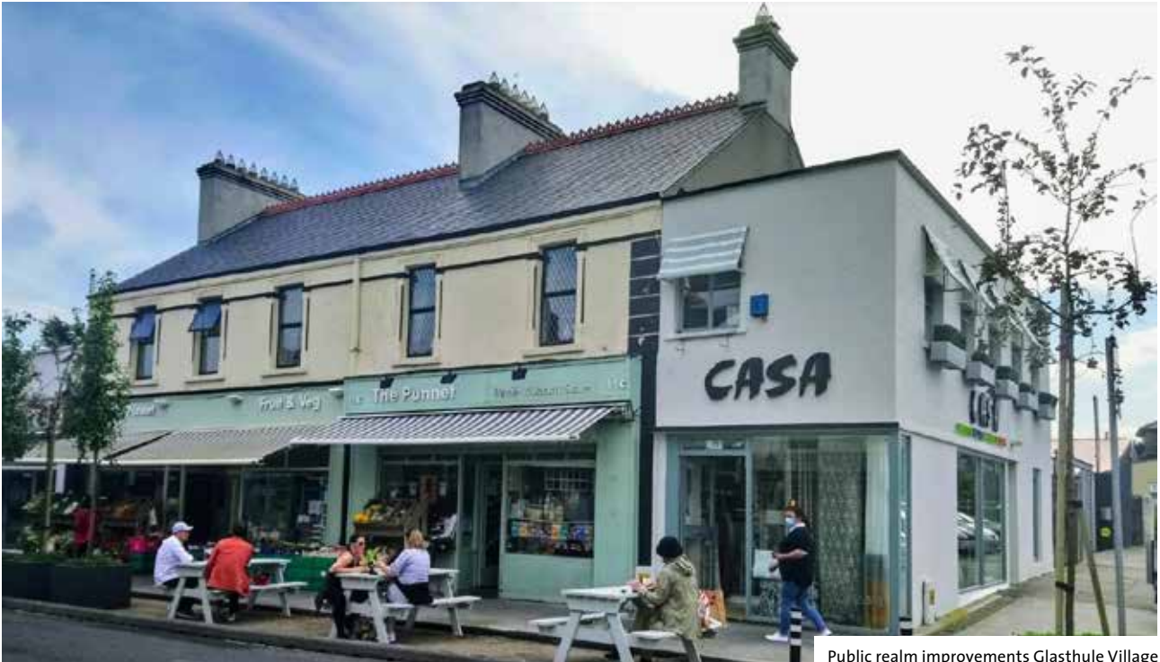
Public realm improvements Glasthule Village
