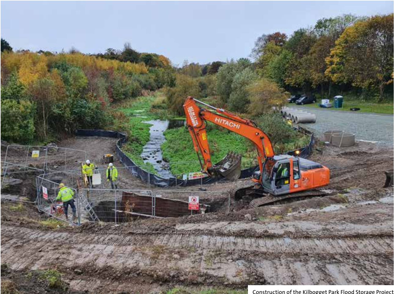
Construction of the Kilbogget Park Flood Storage Project
