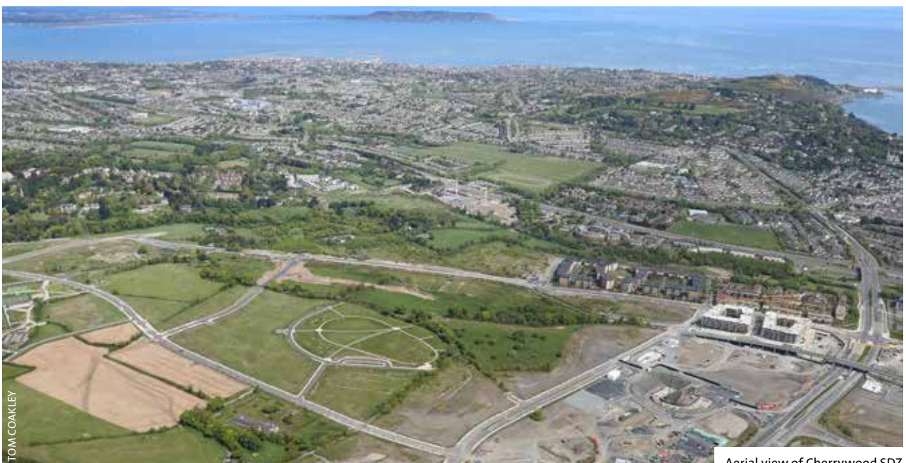
Aerial view of Cherrywood SDZ
