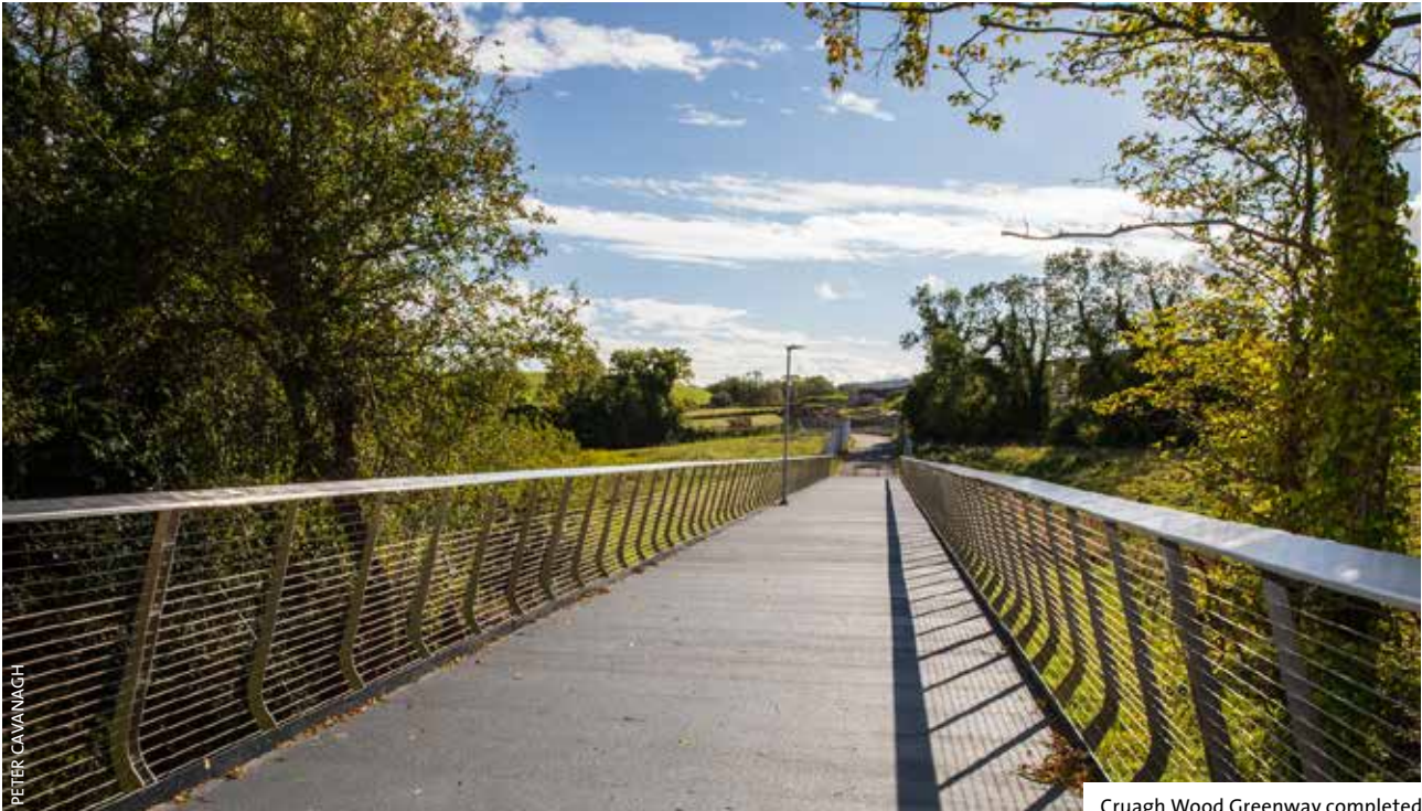
Cruagh Wood Greenway completed
