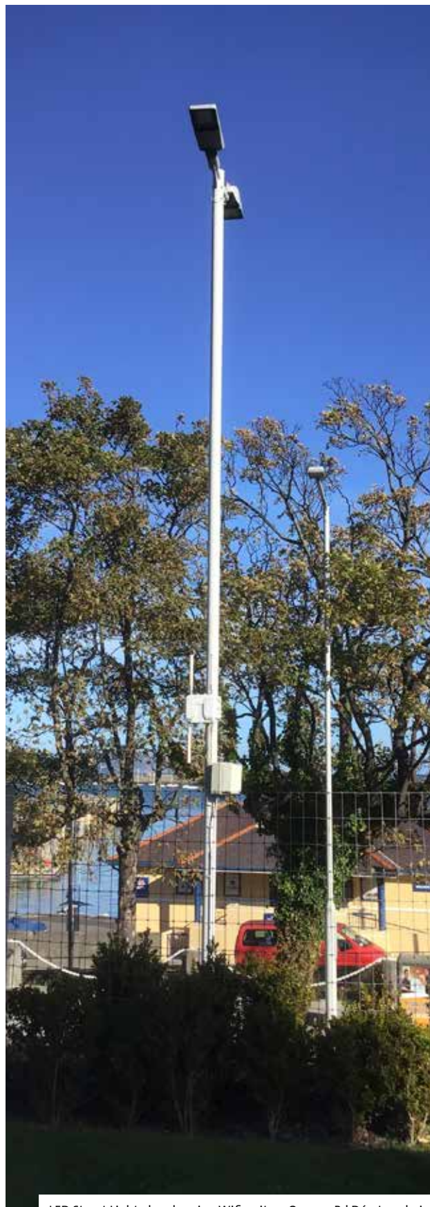
LED Street Light also showing Wifi unit on Queens Rd Dún Laoghaire
