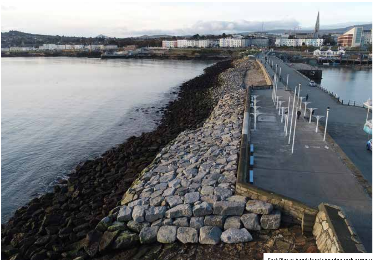
East Pier at bandstand showing rock armour
