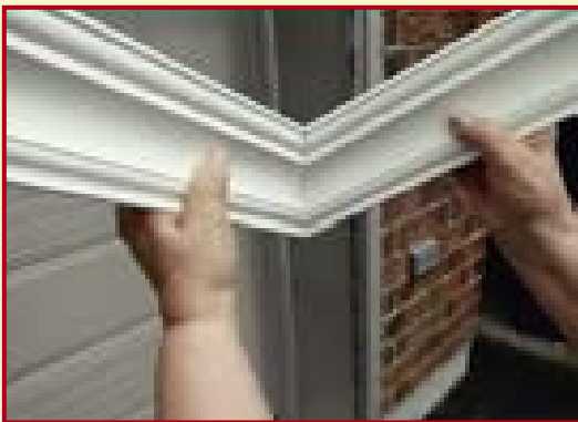
Create perfectly fitting interior crown molding joints
