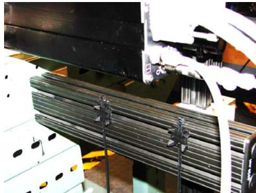
INSERT TIE WRAP MOUNT IN BAR AND TURN 90°. INSERT TIE WRAPS INTO MOUNTS.
