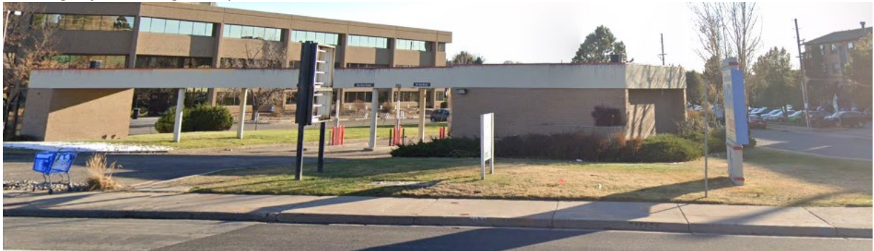
Subject site facing south from Leetsdale Drive
