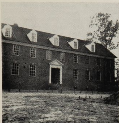
Front of Butler's new Shelter nearing completion.
