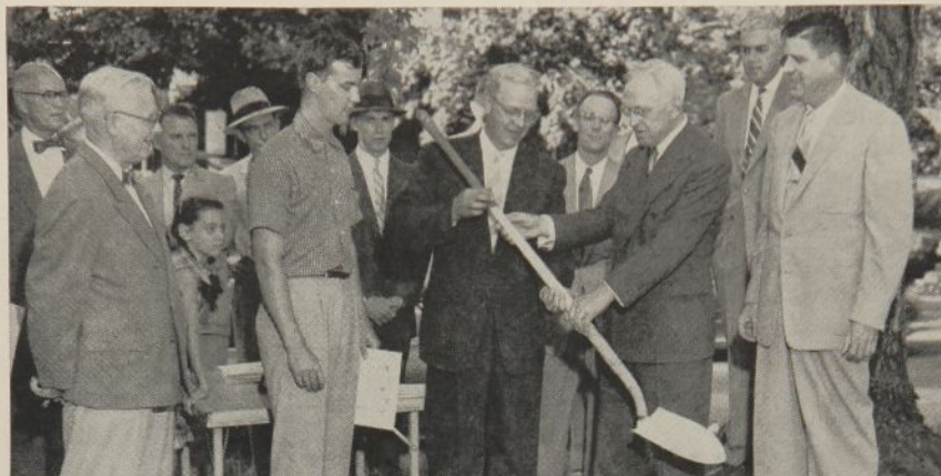
GROUND-BREAKING CEREMONIES involved these principals: Left to right: DOWNIE MOORE, architect; TOM LANE, president of Beta Phi Chapter; KENYON CAMPBELL, house corporation official; WALTER HEER, JR. (looking over Mr. Campbell's shoulder); GEORGE SHOEDINGER; and JAKE SHAWAN, house corporation president.
