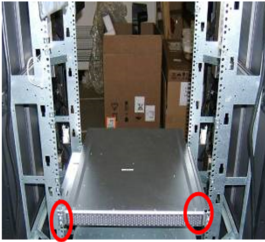
Figure 31 Top rail bracket attachment
