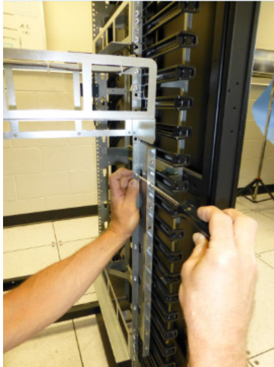
Figure 57 MDS9700-cabkit installed in lower cabinet position.
