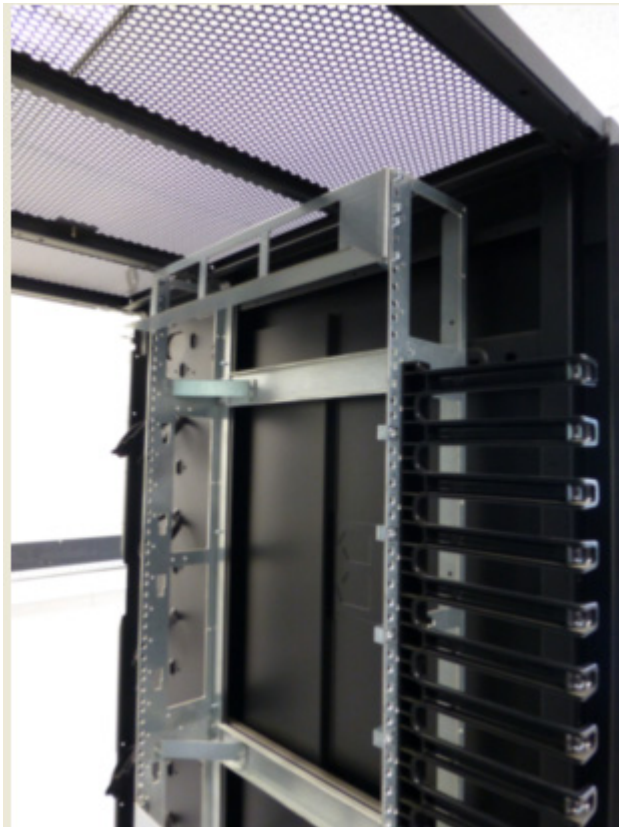
Figure 59 Upper left shelf bracket and clip nuts
