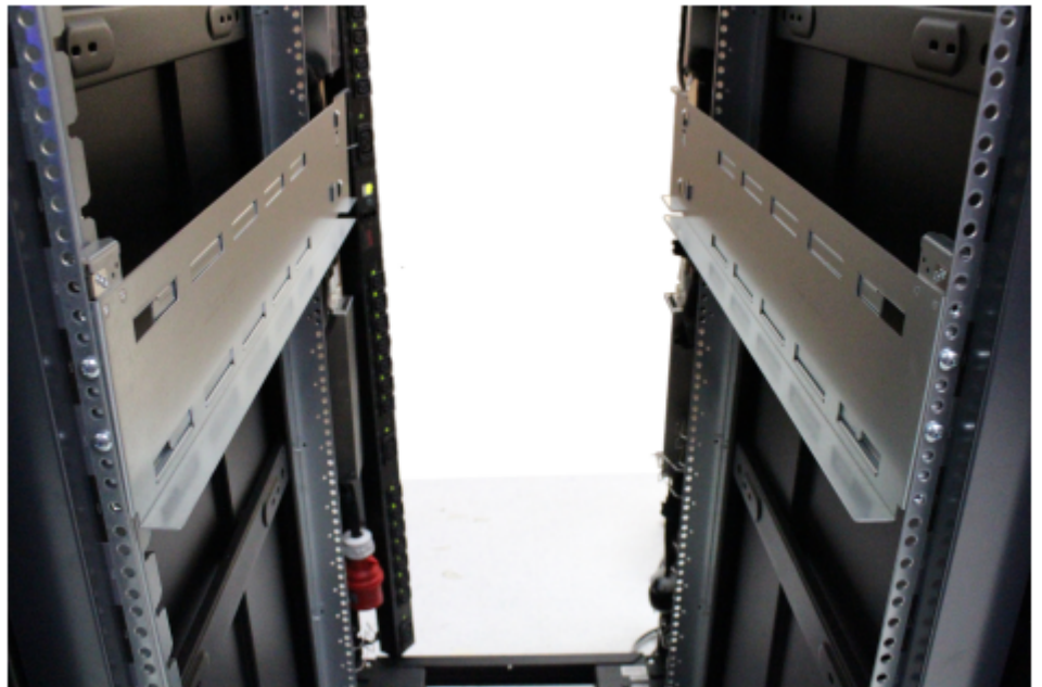
Figure 24 Attach bracket to front of rack
