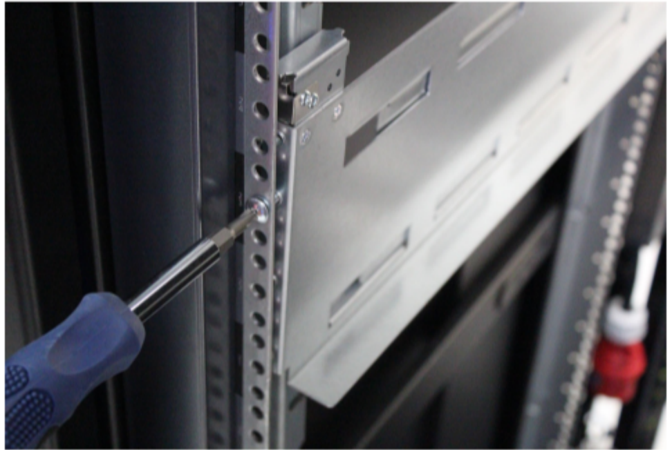
Figure 23 Insert screw in the front
