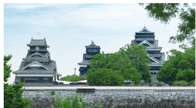
Kumamoto Castle, damaged by the earthquakes (photo from the Ninomaru Parking Lot)
