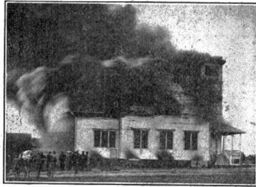
AFTER THE FIRE
