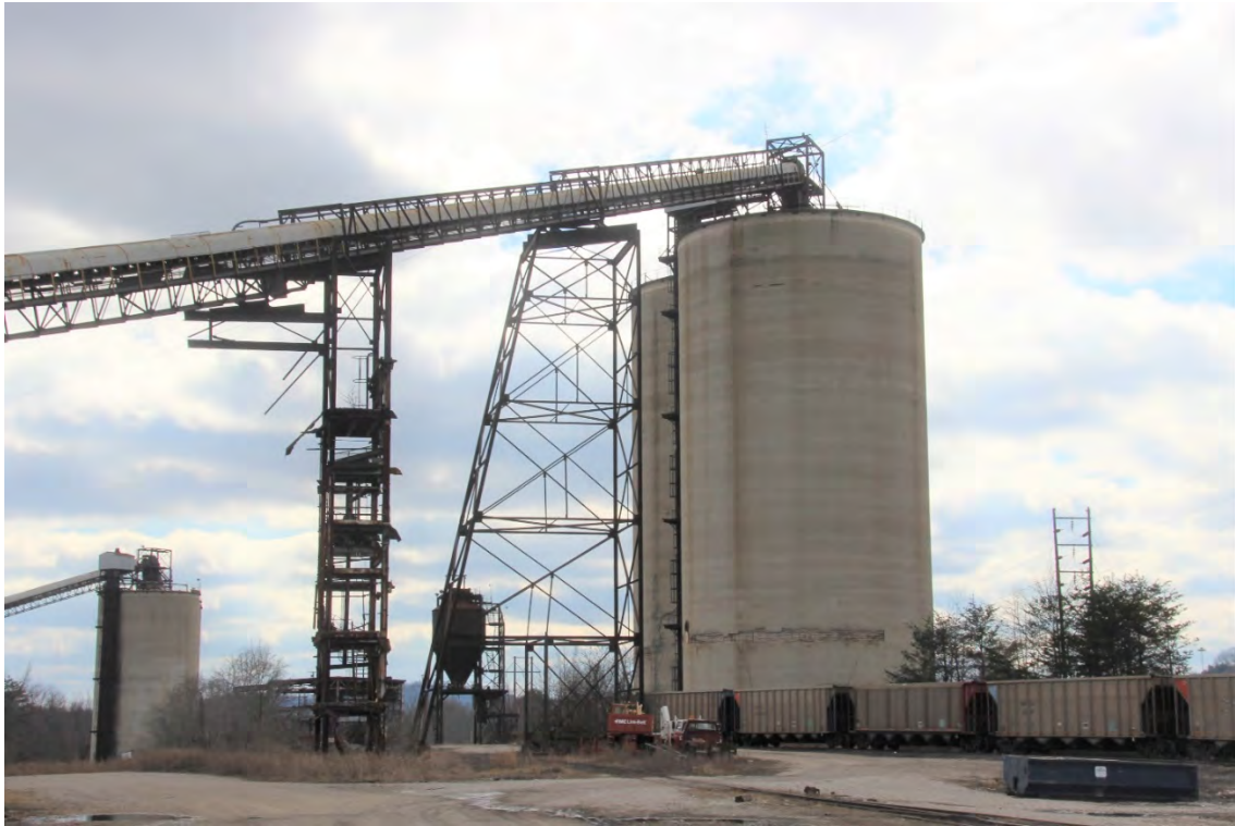
The main coal wash plant. The hopper cars are in storage.
