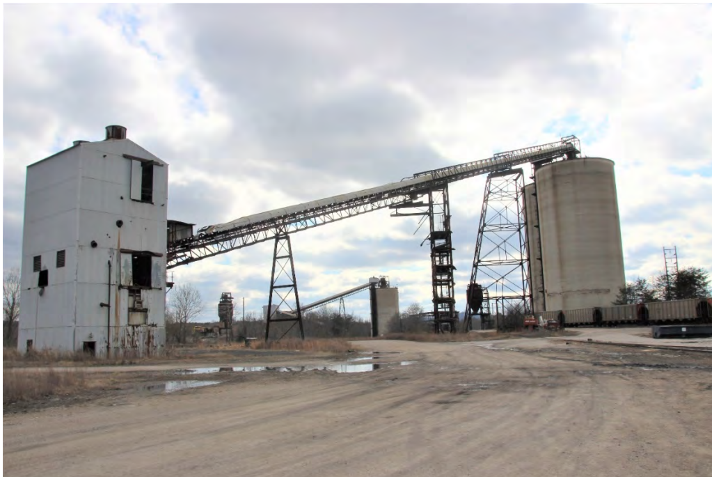
A general view of the remains of the coal preparation plant. The hopper cars on the right were in storage.
