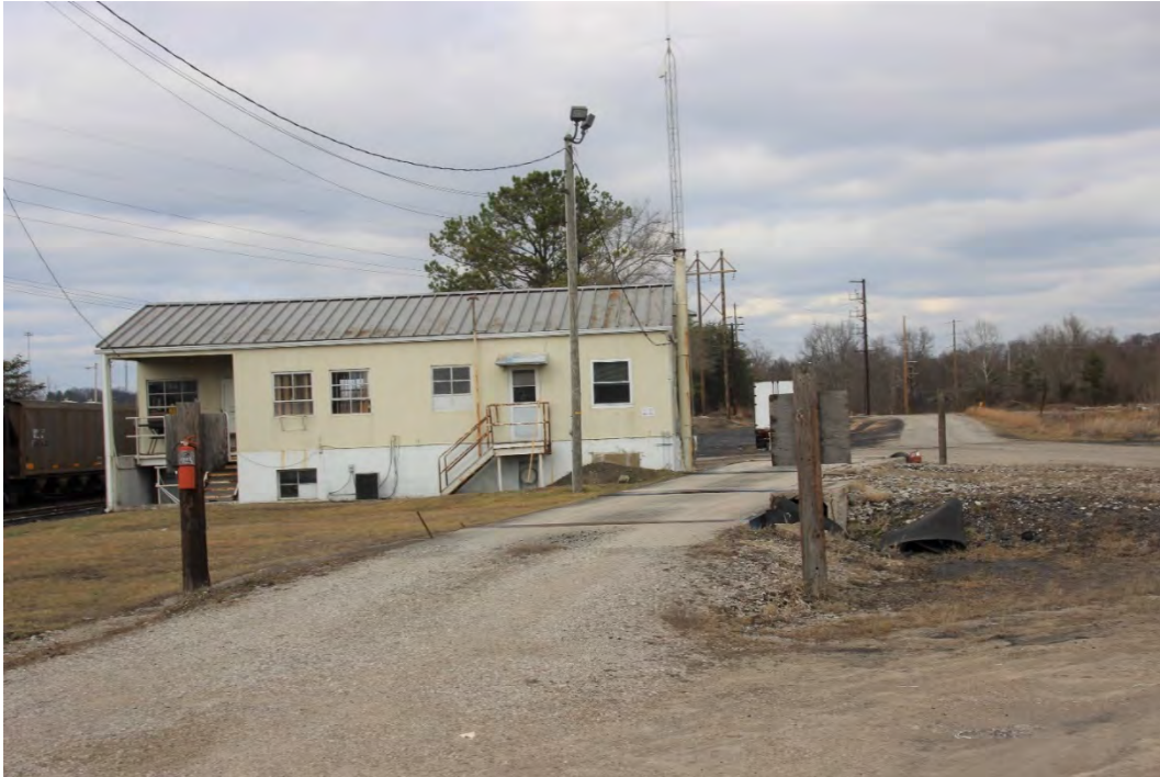
This building was being used by ARQ as their local office.
