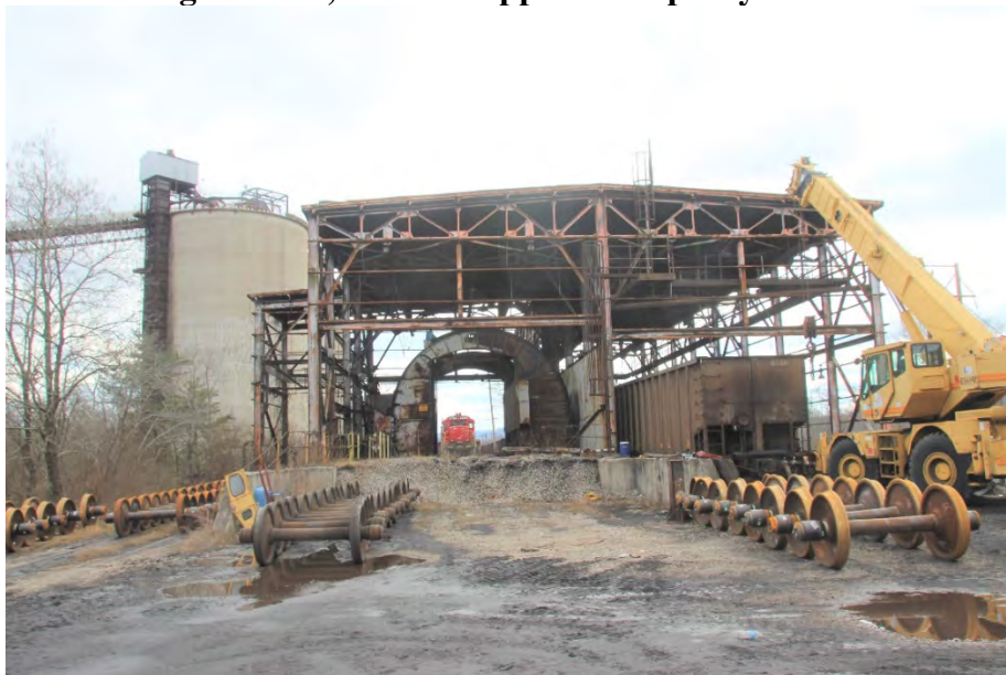
A view of the hopper repair car area. The Progress Rail locomotive is framed by a rotary coal car dumper.
