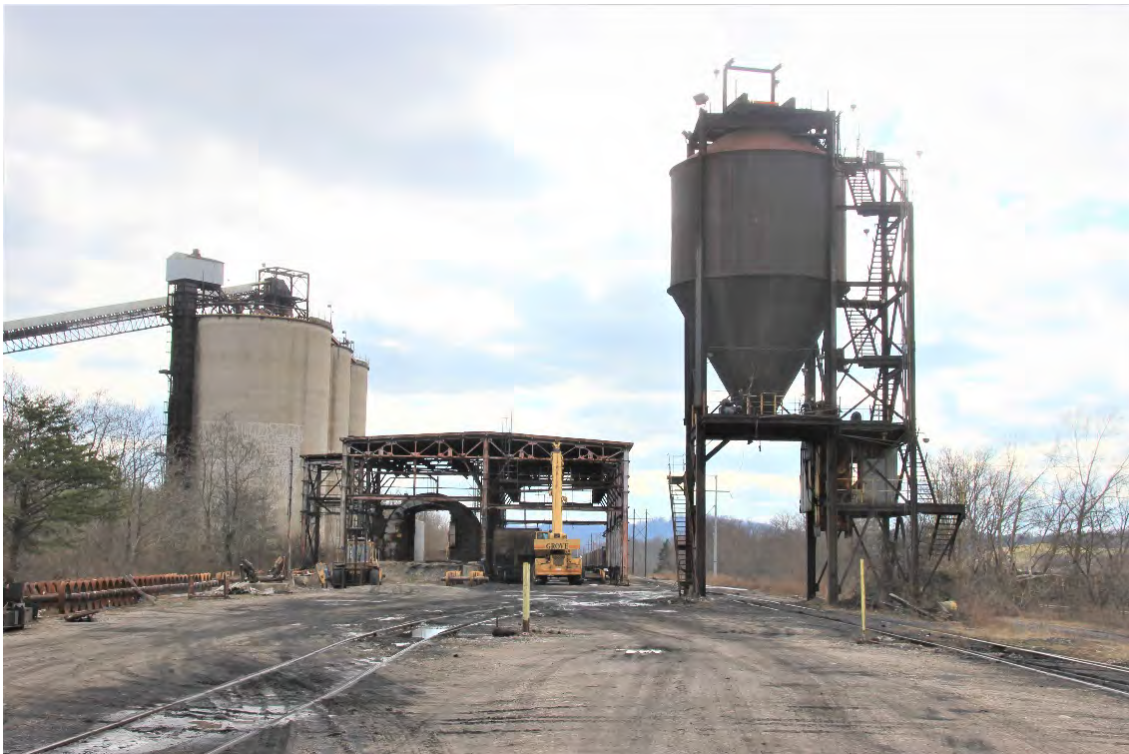
What is left of the US Steel railyard at the wash plant. A rotary dump can be seen in the left bay of the building in the center
