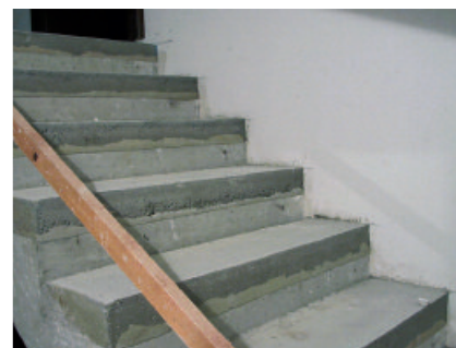
Due to its properties, PCI Novoment M3 plus is also suitable to compensate the height of concrete steps.
