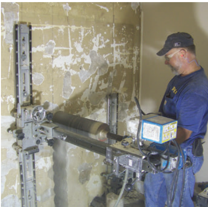
Drilling a line of holes using the stitch drill.
