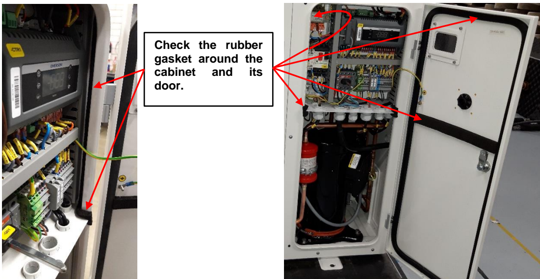
Figure 36: Visual inspection of the rubber gasket
