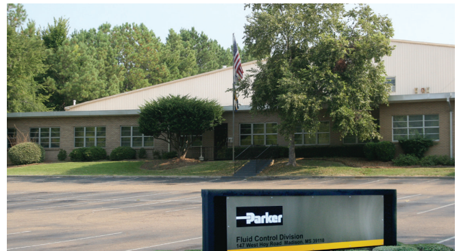
Fluid Control Division Facility, Madison, MS.
