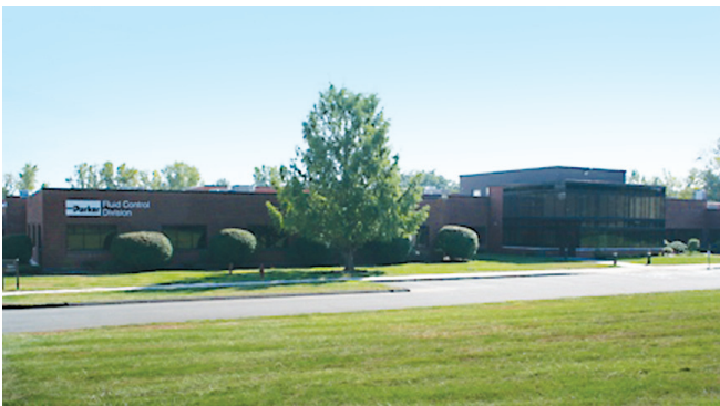
Fluid Control Division Headquarters, New Britain, CT.
