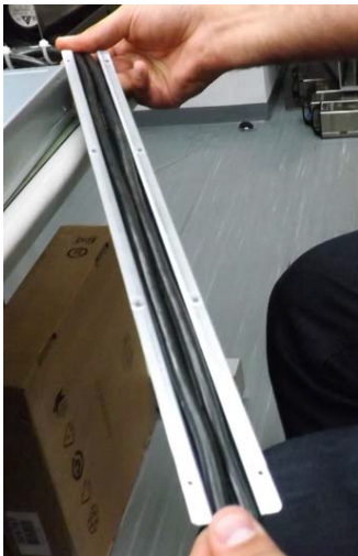
Cables within the Rail
