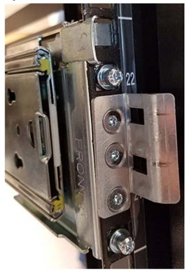
Figure 26: Rack Latch Bracket Installed
