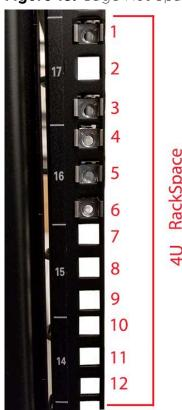
Figure 18: Cage Nut Spacing
