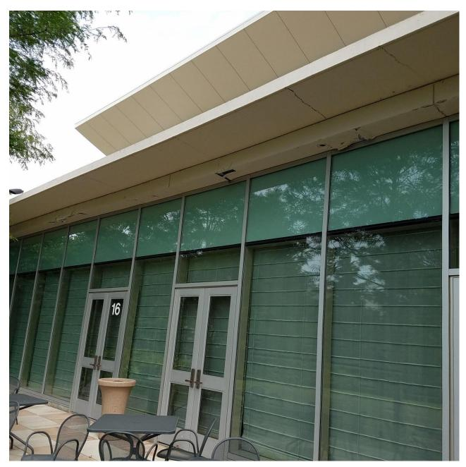
This photo represents the soffit degradation at the cantilevered roof section above the Waterleaf restaurant. The protective coating on the concrete roof slab above has been compromised due to (non-structural) concrete cracks that have developed since constructed. This project seals the cracks, provides a 20 year waterproof membrane reinforced roof slab coating and repairs the water damaged soffits.
