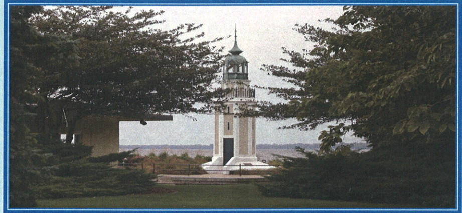
Buckstaff Lighthouse - Bayshore Drive - Oshkosh
