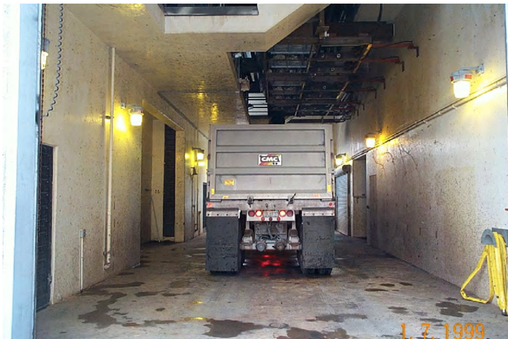
Photo 2 - Truck beneath biosolids hoppers
