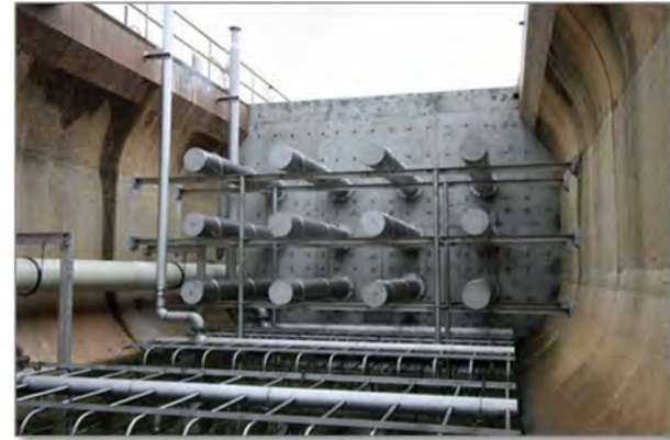
Baffle wall with media retention screens
