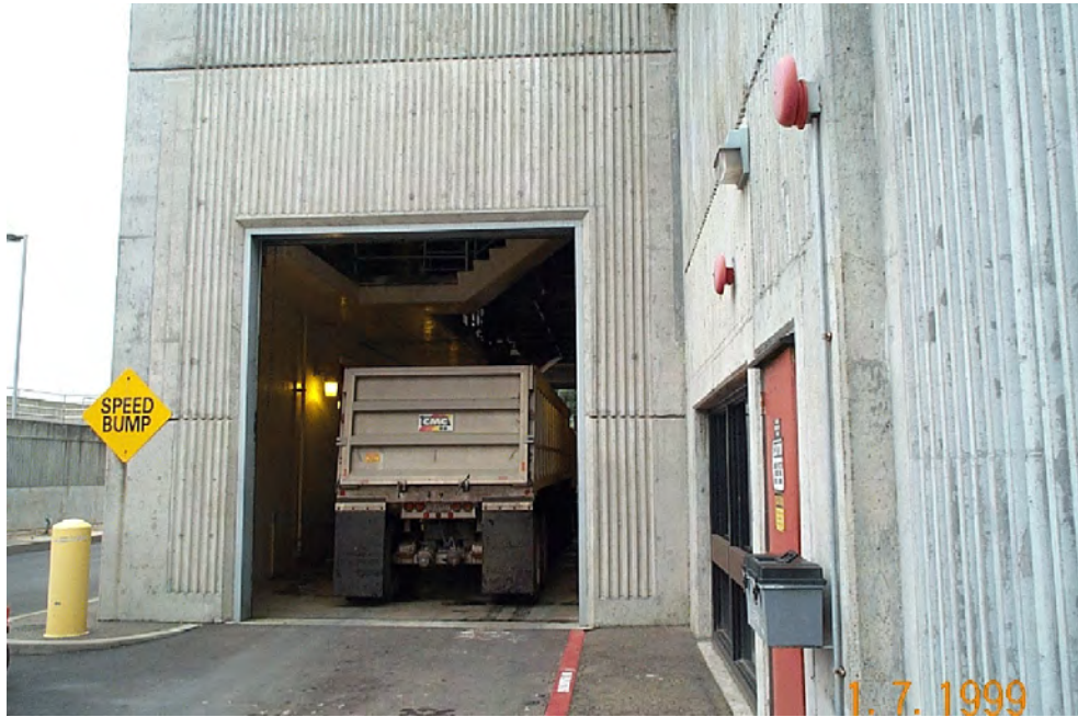
Photo 1 - Truck entering solids handling loading bay
