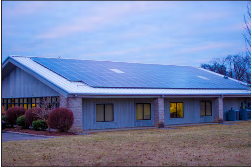
Photo Courtesy of Mid South Construction
