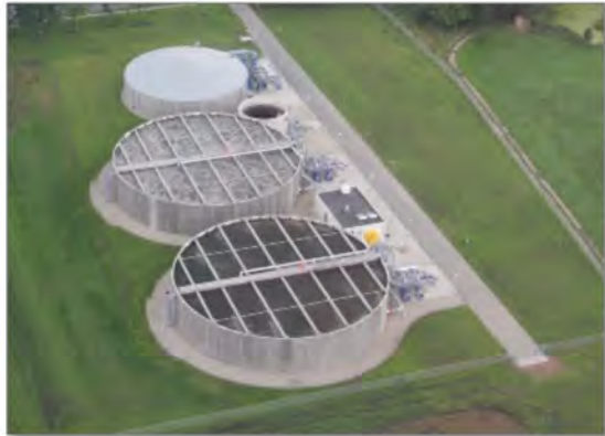
AGS reactors in react/aeration mode (top) and settle mode (bottom)
