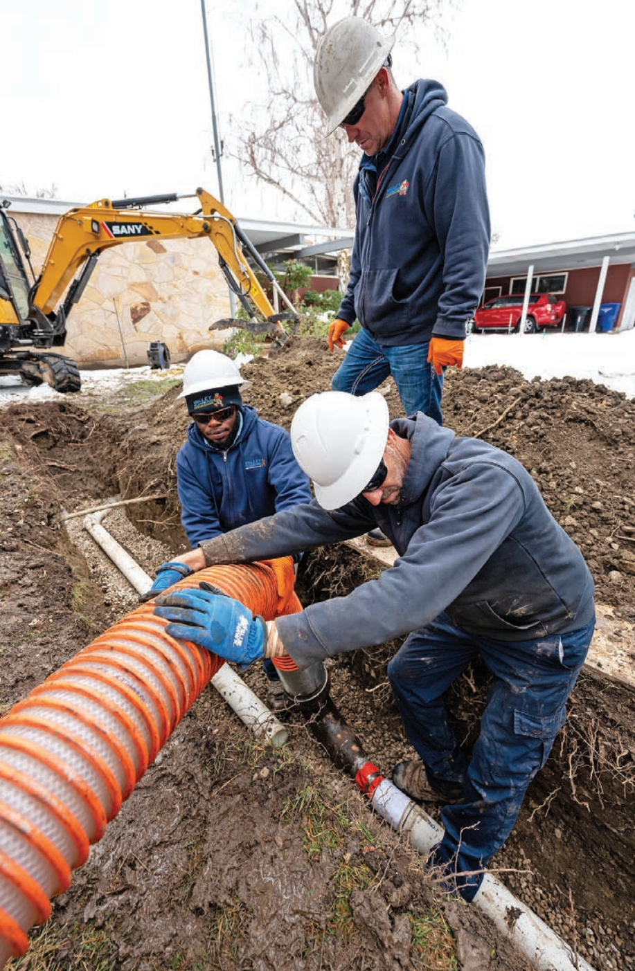
➤ Jules Matabishi, excavation manager Michael Sides and Joey Howard (from left) move a loaded lining system into position.
