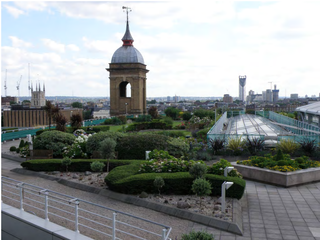
Picture 4: Cannon Bridge House
