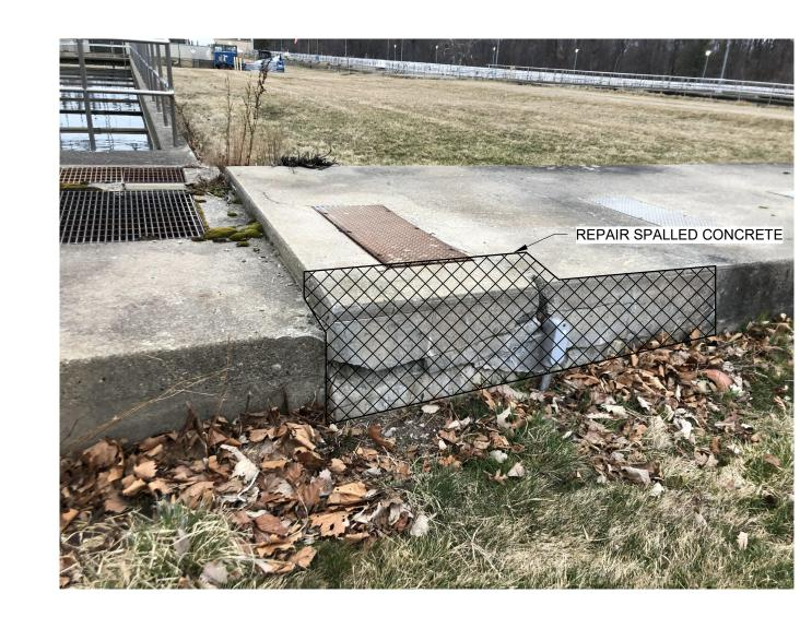
REPAIR TOP SLAB OF PIPE GALLERY AT PRIMARY SETTLING TANK
