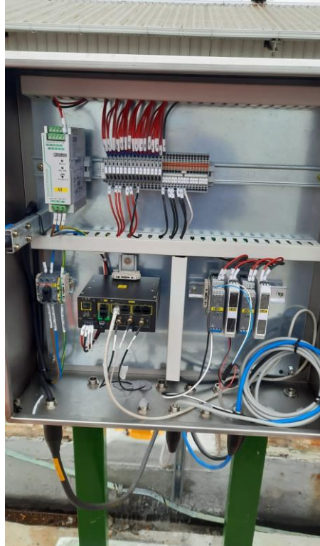
NEMA-4X Enclosure with IR, and I/O terminal blocks
