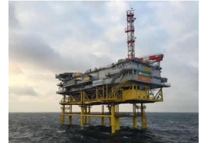
Example: Offshore Substation (OSS)
