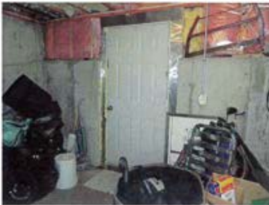
Bulkhead Entry / Exit Basement
