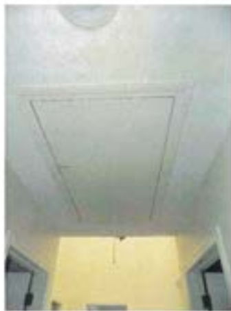
Attic Pull Down Access Hallway Second Floor
