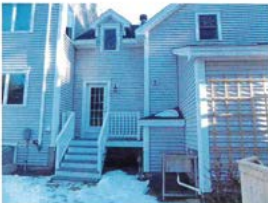
Outdoor Sink Rear of Subject
