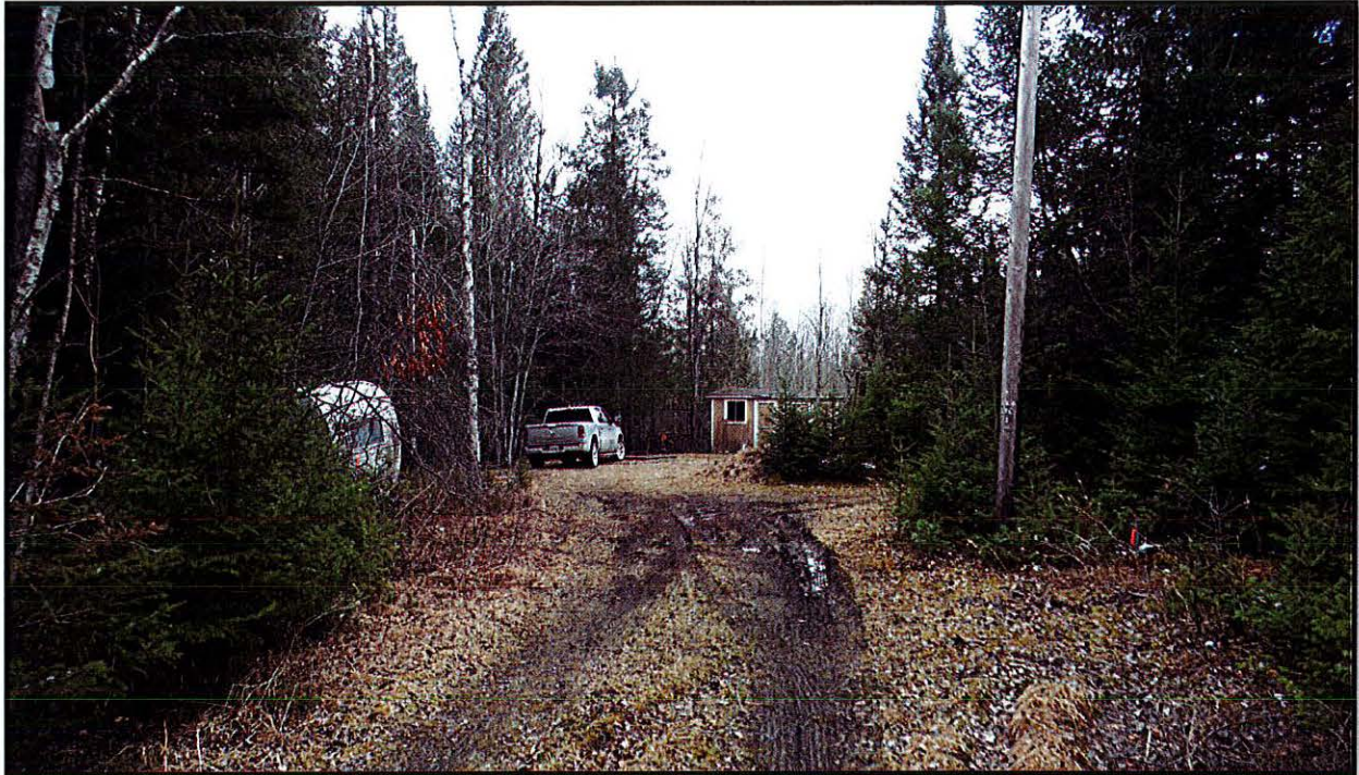
Figure 1. Location of subject property at 515 Englewood Lane, Ellis Twp. (Existing shed visible in center of photo).
