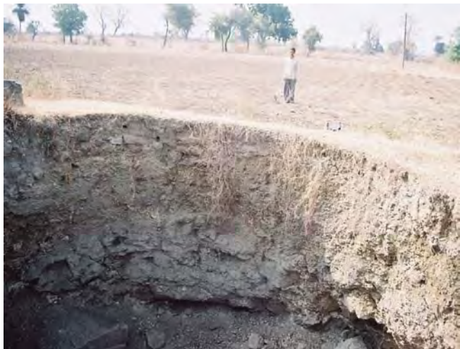
Collapsed well in farmers field at Chikmoh
