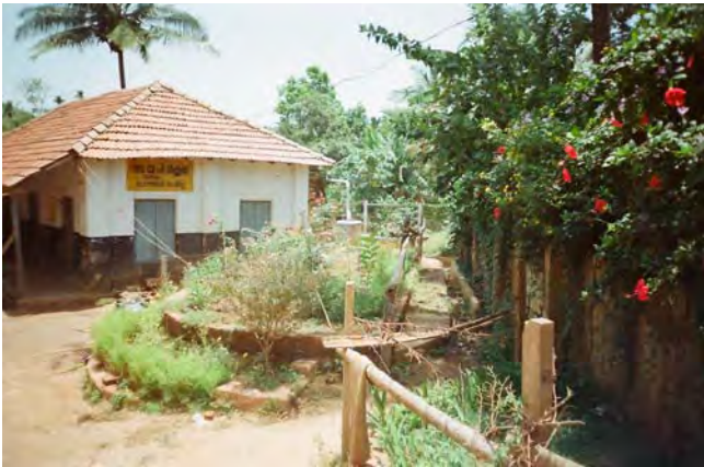
Rain water Harvesting in Government UP School, Thalapuzha, Wayanad District. Rainwater collected in surface tank and flowers planted over the tank. The structure constructed with the financial support of MOWR
