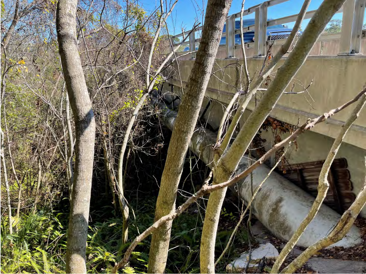
Looking Downstream at north end of Lake Bosse Bridge
