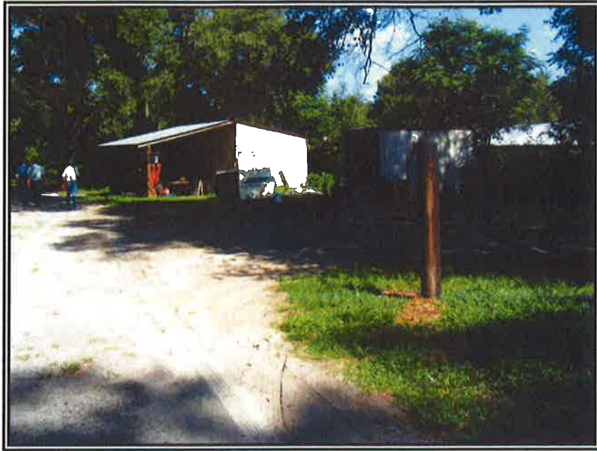
3. LOOKING NORTHWEST AT THE STORAGE SHEDS
