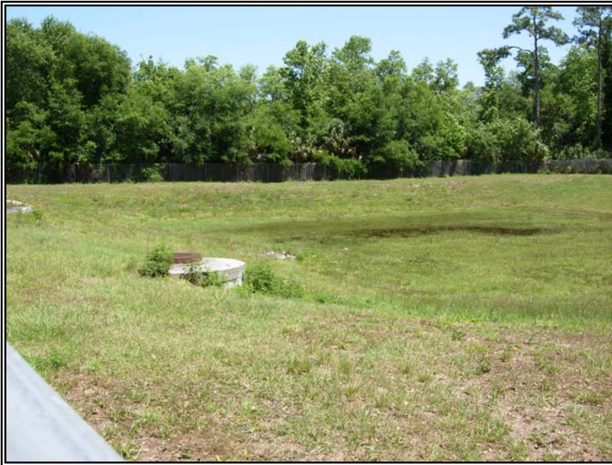
Photo 18: Representative photo of the existing FDOT in the area of Pond 3 and 3A
