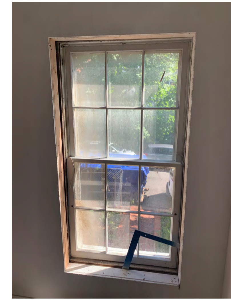
MAIN LEVEL RIGHT FRONT WINDOW
