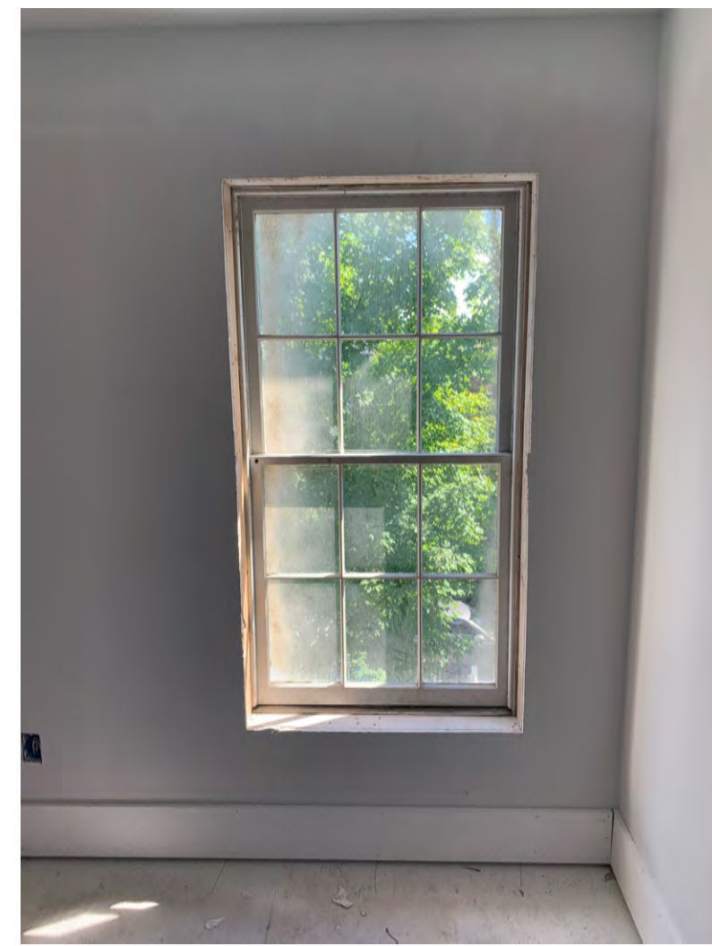
UPPER RIGHT FRONT WINDOWS
