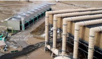
**3. Hybrid cooling** (wet and dry) is illustrated conceptually at the left, in service at right
