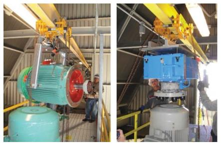
**10. Low-profile lifting devices** are used to remove fan motor drivers and gearboxes
