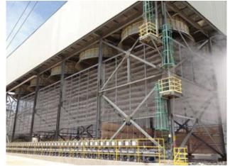
**12. Fogging system** installed at Midlothian to demonstrate performance improvement increased steam-turbine output by 5.8 MW at 100F and 30% relative humidity
