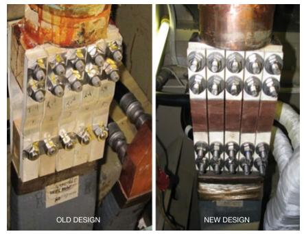
9. Replacement connection rings (right) feature double the number bolts on the lower tang compared to the original five-bolt design at left
