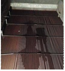
**12. This leak was found** by filling the reheater with water via RH attemperator sprays
