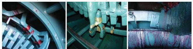
35. Repairs to vibrating components included replacement of connection-ring ties
