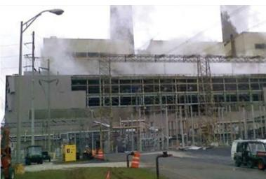
**45. Siding was blown off plant exterior** by the detonation wave that occurred because of inadequate hydrogen purging procedures
