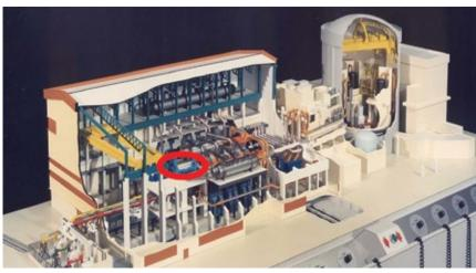
**48.** Powerplant model shows the revenue machine (generator, encircled by red ellipse) virtually hidden by other equipment
