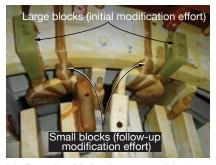
**28. Repaired joint** features added support stiffness to increase phase-bar natural frequency
