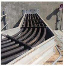
3. Long-lived spacers of high-density polyethylene were installed without incident
