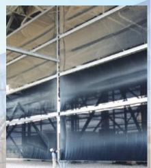
Top: Wind deflection screen Bottom: Wind and dust control fence showing integration of a doorway and conveyor
