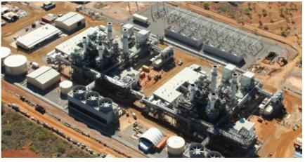
**5. Diamantina Power Station,** which produces 240 MW with two  $2 \times 1$  power blocks, took steps to reduce dissolved oxygen in cycle water
