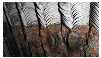
7. These tubes had been frozen and damaged by debris trapped behind support beams
