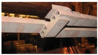
20. Detail of original connection is revealed during disassembly
