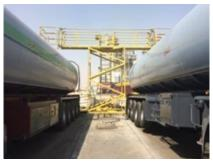
**1. New platform,** designed by plant staff, serves two oil tankers simultaneously
