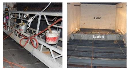
7. Scaffold at left is prepared for duct-burner baffle-reinforcement at right
