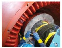
36. Generator rotor end plate before inspection
