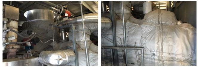
**Blankets for heating** the HP cylinder (left) and crossover (right) to enable faster starts **COMBINED CYCLE** JOURNAL, Number 51, Fourth Quarter 2016
