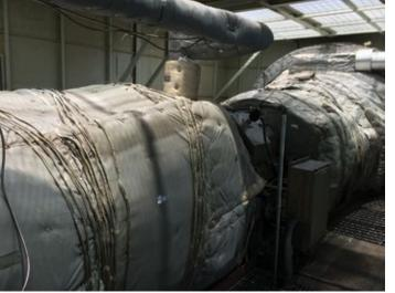
A10 steam turbine has heating blanket to enable fast starting
