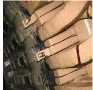
**40. Mechanical vibration** contributes to insulation degradation
