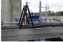
**2. Cable lifting rig** was designed and fabricated by plant personnel
