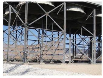
**11. Placement of ground-level screens** was based on results of CFD modeling
