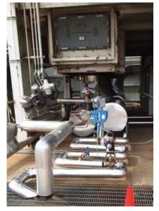
6. Problem solved with new automated drain line and addition of access doors
