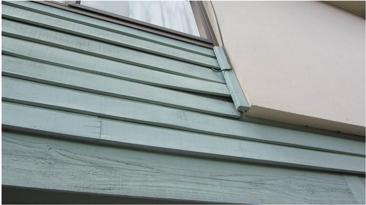
Photo 23: Timber wall cladding on Block B.
