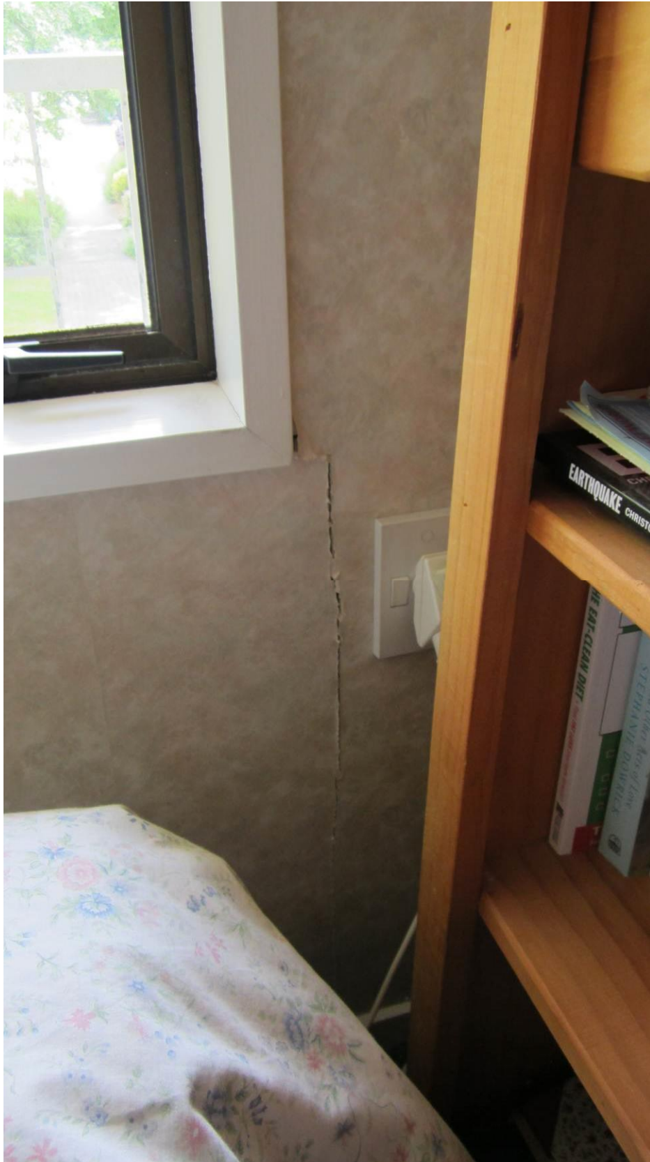
Photo 19: Internal wall linings.
