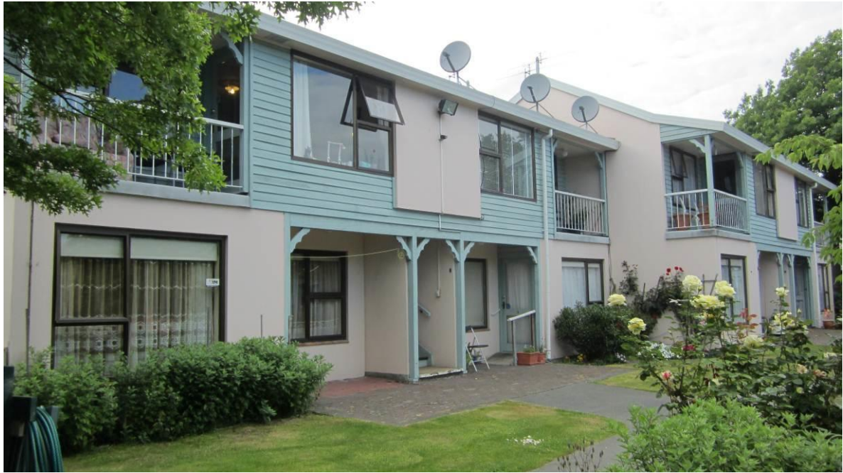
Photo 1: External view of Block A from north-west.
