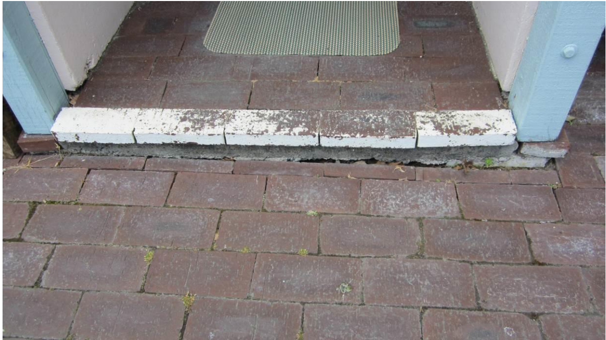
Photo 9: Typical paving at front of Block A and Block B.
