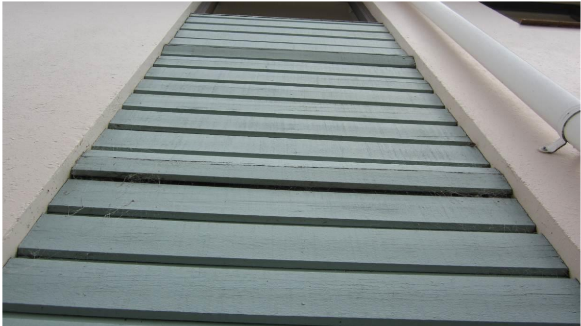
Photo 24: Timber wall cladding on Block B.
