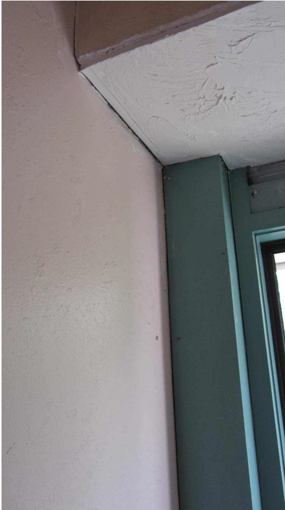
Photo 18: Typical internal wall and ceiling linings.
