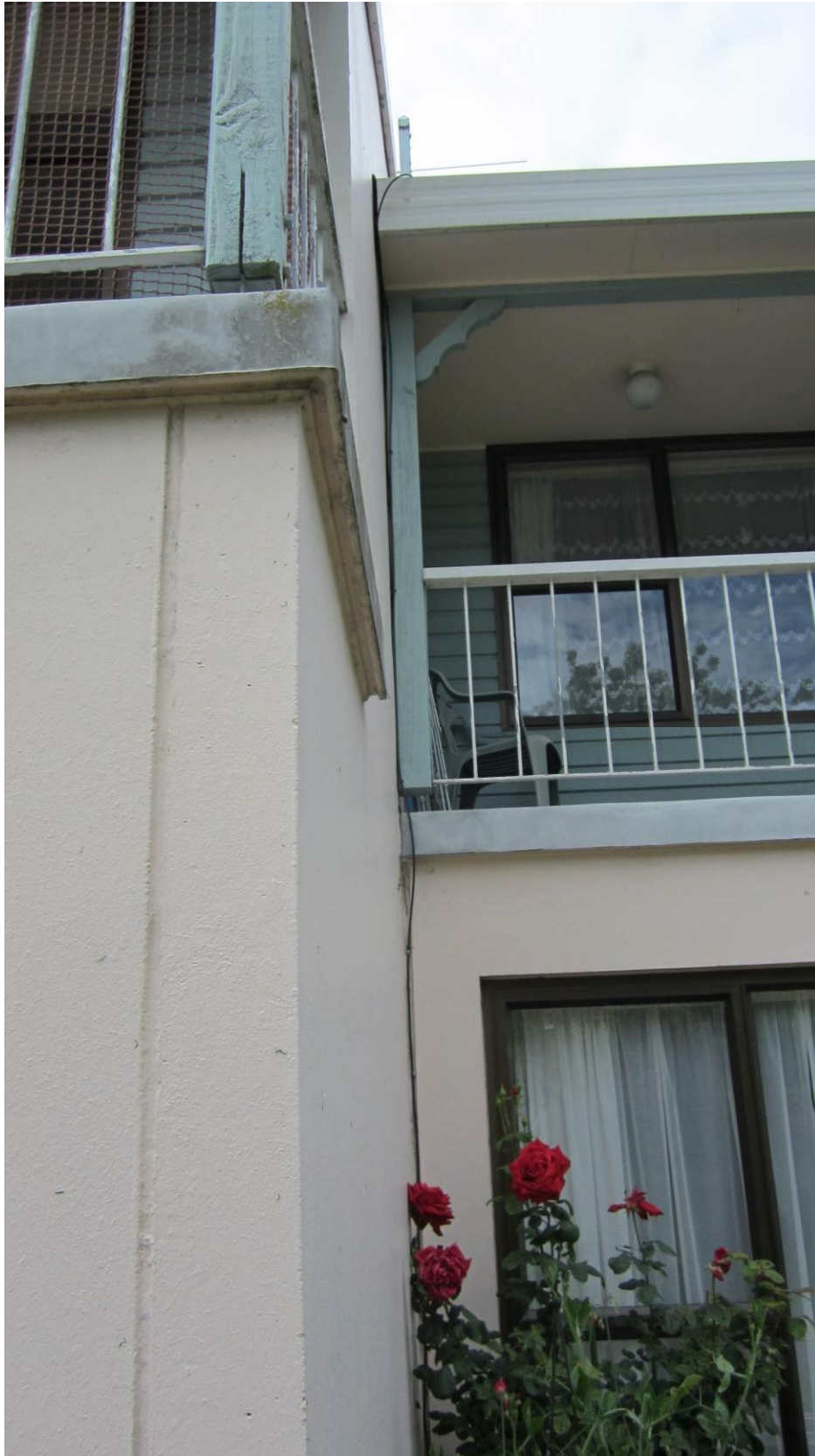
Photo 21: Centre precast concrete wall panel of Block B (view from north).
