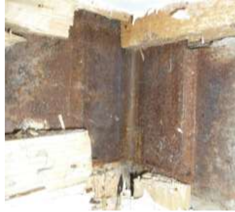
Unit 2 weld plate showing 2 welded sides
