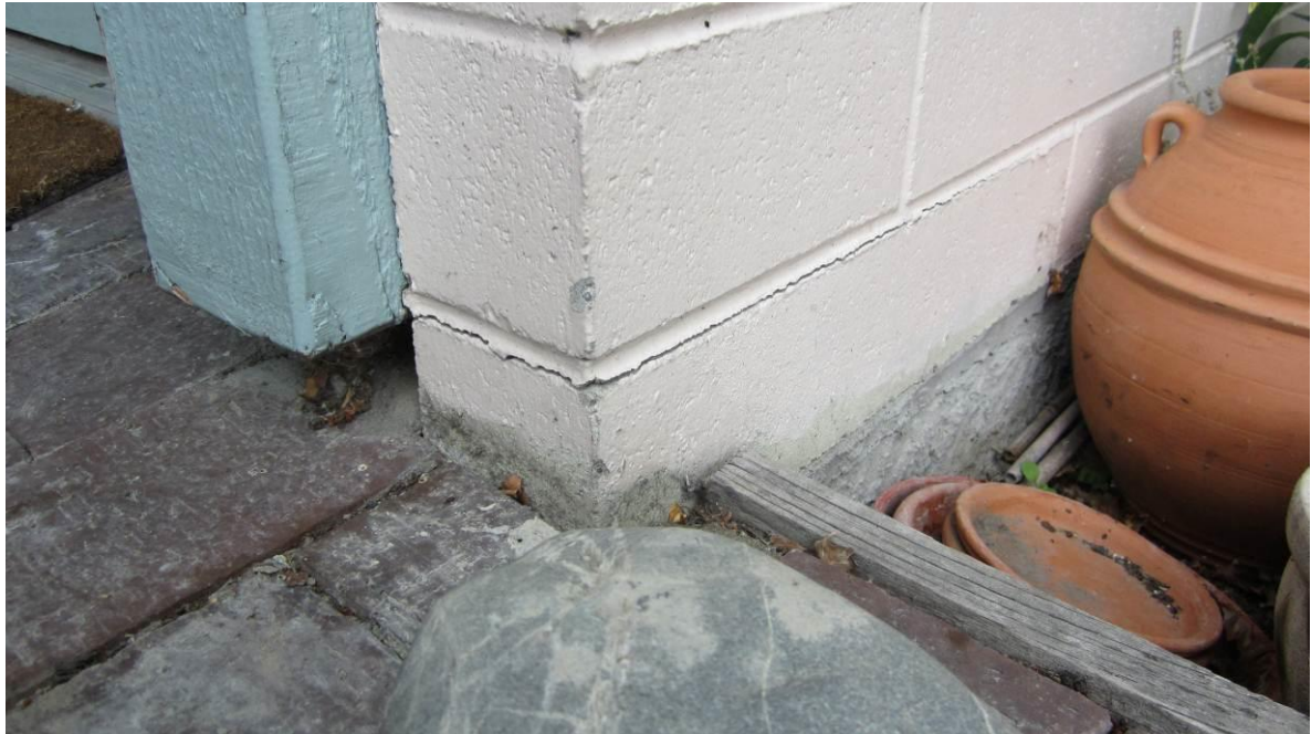
Photo 27: External concrete masonry block veneer at front terrace of Block C.
