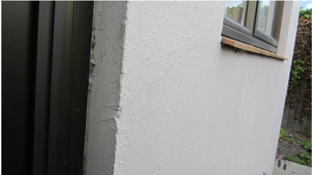
Photo 7: Precast concrete wall panel at rear of Block A.
