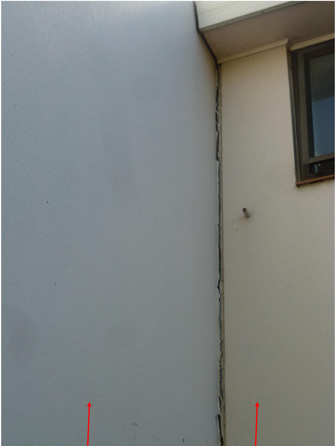
Photo 4: Units 13 & 14 moving away from units 11 & 12
