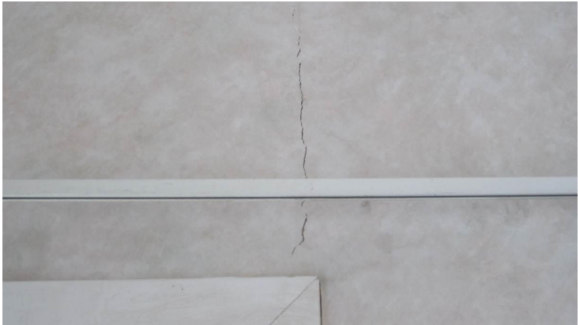
Photo 17: Internal wall linings, typical for all buildings.
