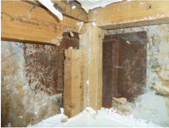
Unit 4 weld plate showing 3 welded sides
