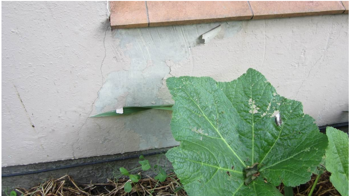
Photo 11: Precast concrete wall panel at end of Block B.
