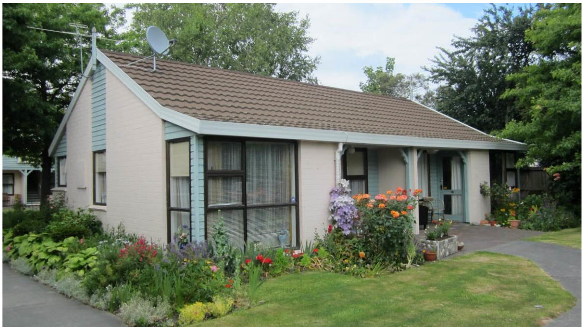
Photo 4: External view of Block C from north-east.
