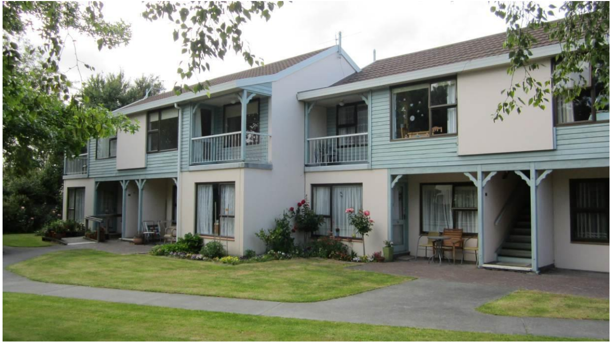
Photo 3: External view of Block B from north-west.
