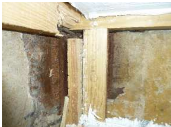
Unit 6 weld plate showing 2 welded sides
