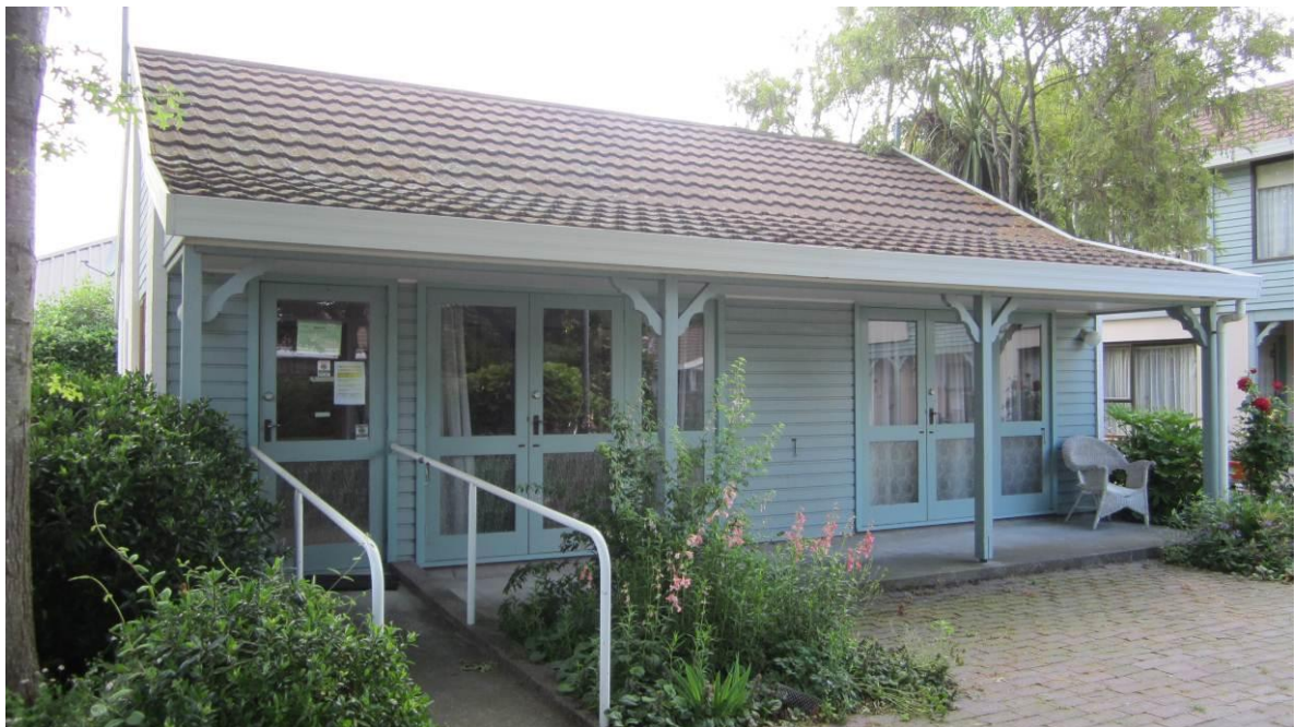
Photo 2: External view of Residents' Lounge from west.
