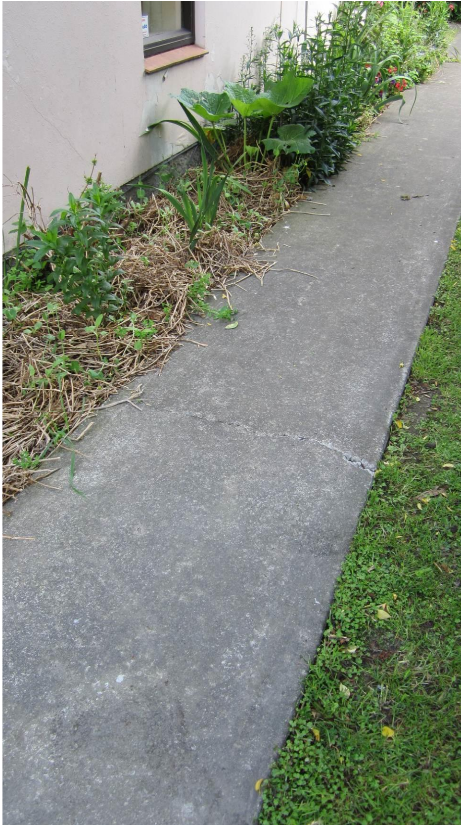
Photo 14: Typical pavement surrounding all buildings.
