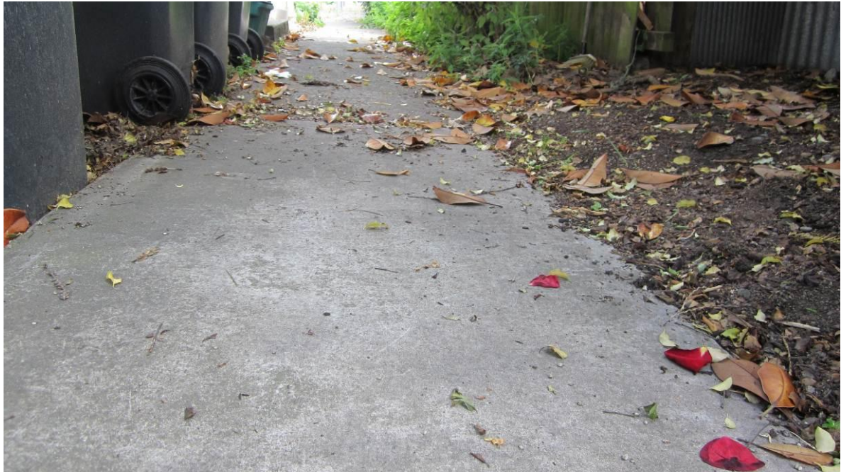
Photo 15: External pavement at rear of Residents' Lounge
