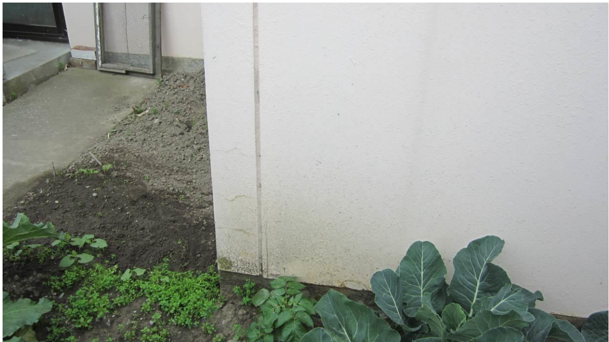
Photo 8: Precast concrete wall panel at rear of Block A.
