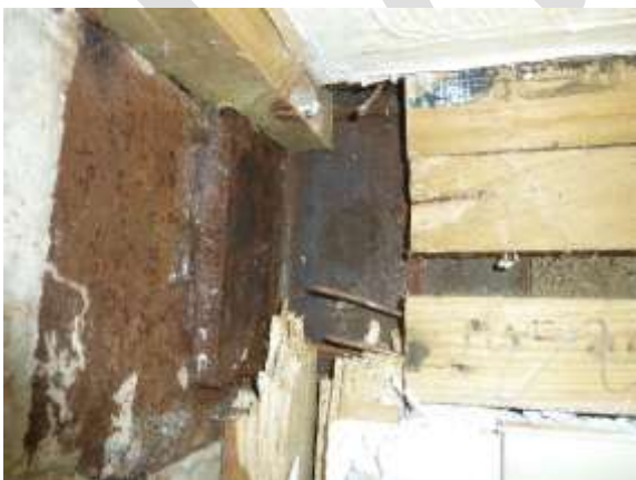
Unit 8 weld plate showing 2 welded sides
