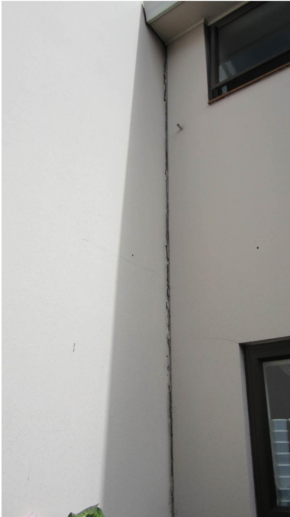
Photo 20: Centre precast concrete wall panel of Block B (view from south).
