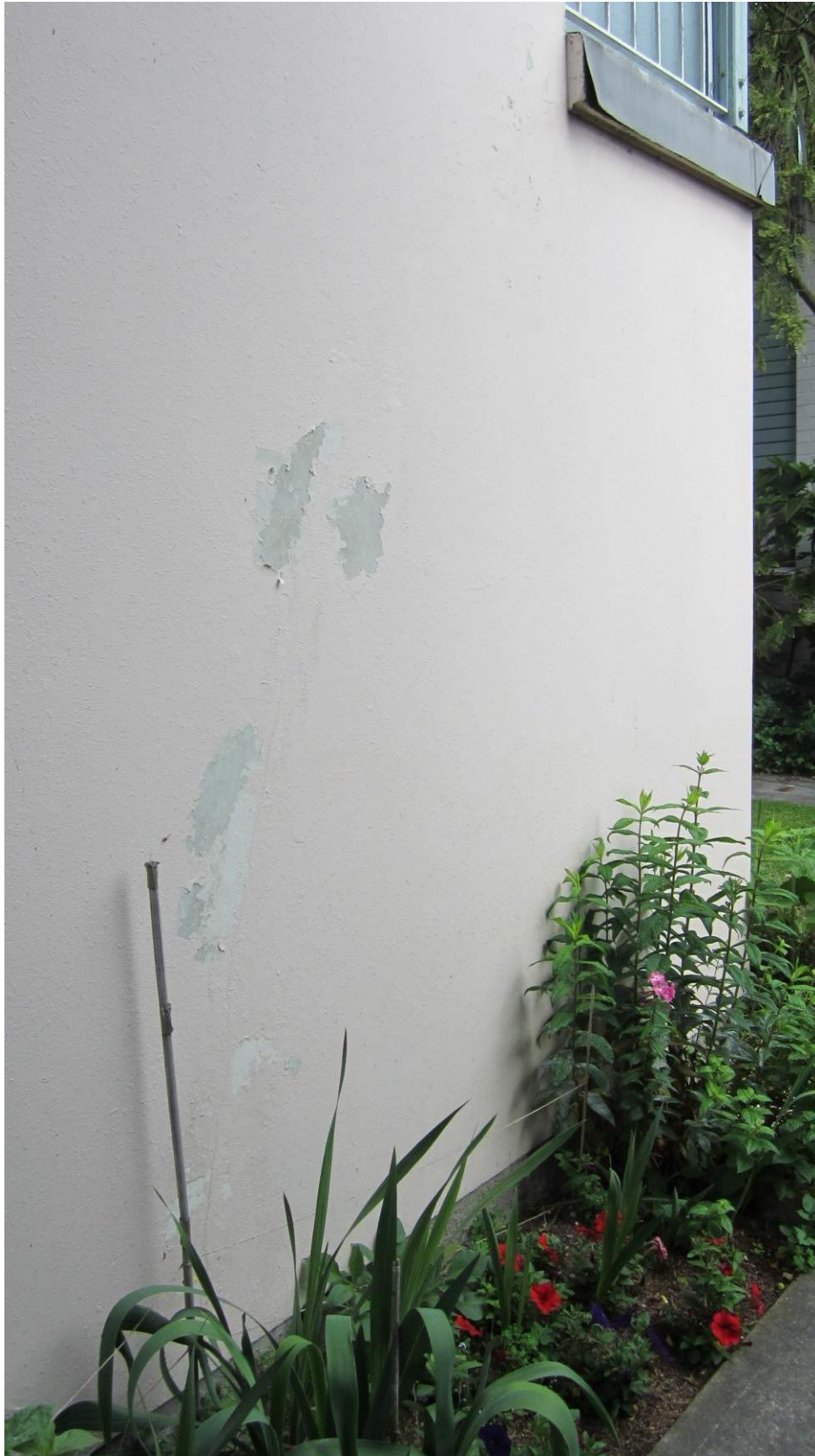
Photo 10: Precast concrete wall panel at end of Block B.
