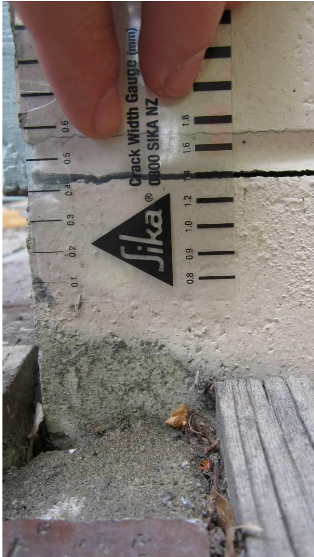
Photo 28: External concrete masonry block veneer at front terrace of Block C.
