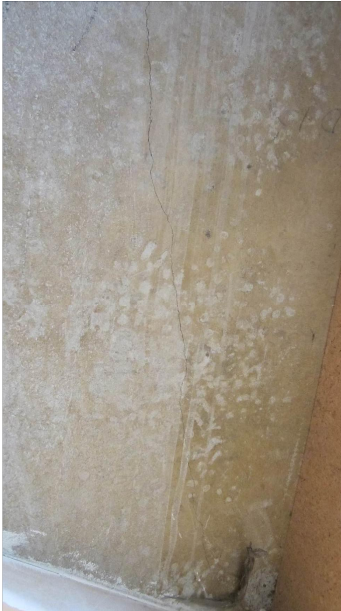
Photo 13: Precast reinforced concrete panel beneath stairs in Block B. (Transverse wall)
