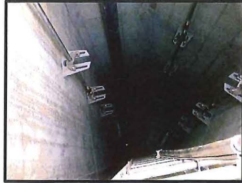
Inside the Completed Junction Structure
