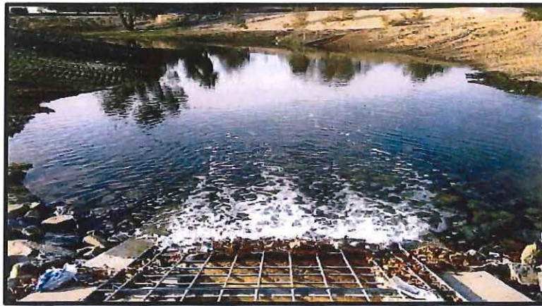
Installed 60-inch connection pipe into Basin 8 Junction Structure
