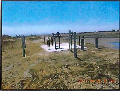
Construction of Junction Structure
