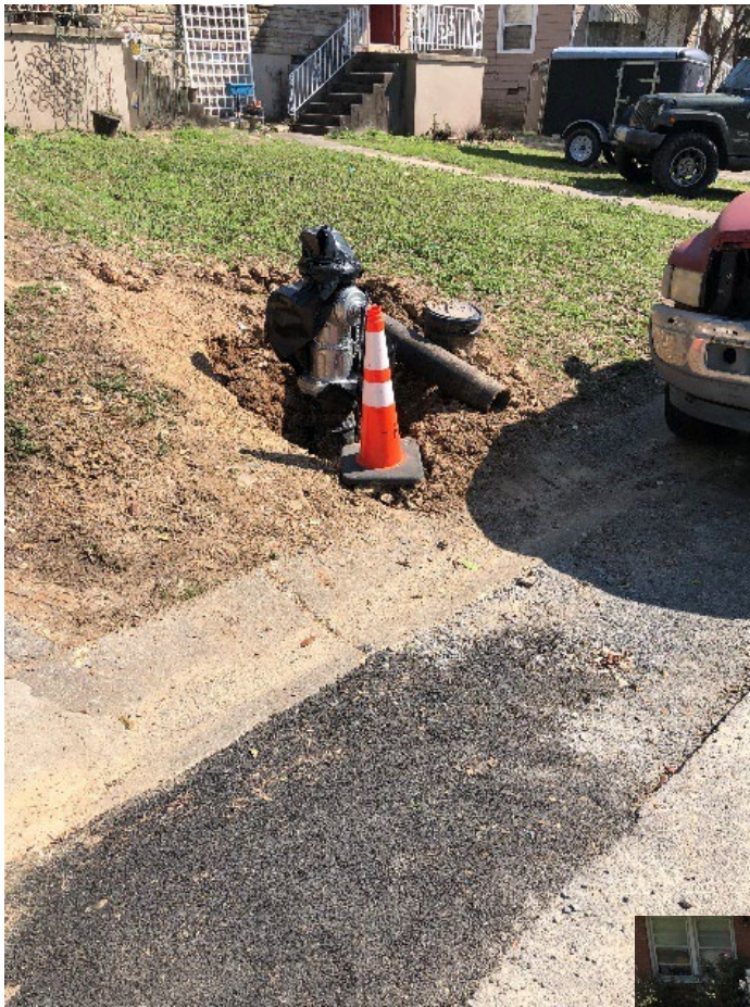
New fire hydrant being added mid-block.
