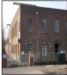
Local Exchange Or BNG Site
