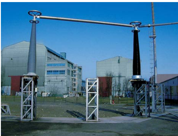
Test Setup of Prequalification Test
