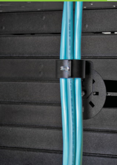
Rack-Mount Universal Clamp Kit Installed
