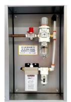
Air pressure affects the ability to draw a high vacuum. We recommend a pressure setting of **85 PSI while the dryer is resting idle**. Air is used when the **vacuum generator** is running so observe the PSI while the Dryer is drawing a vacuum. The gauge should continue to read this setting even when the vacuum unit is on. If it does not maintain pressure your supply line is not sized properly.
