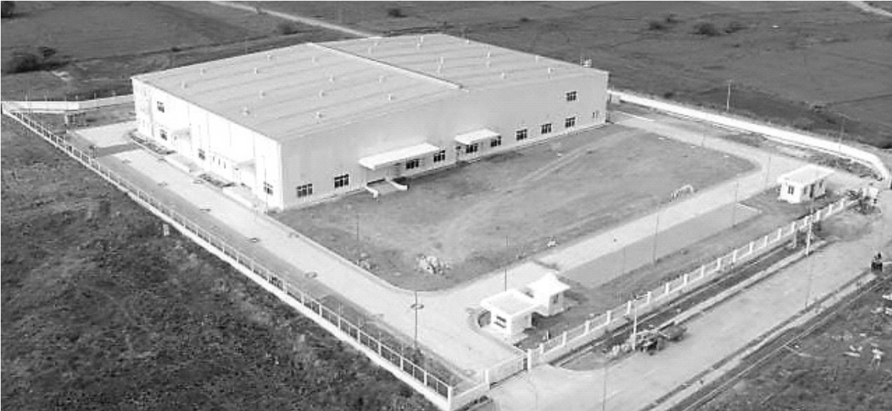
MASL Factory Building For M/s Systematic Conscom Limited at kanchipuram Near Chennai, Tamil Nadu.
