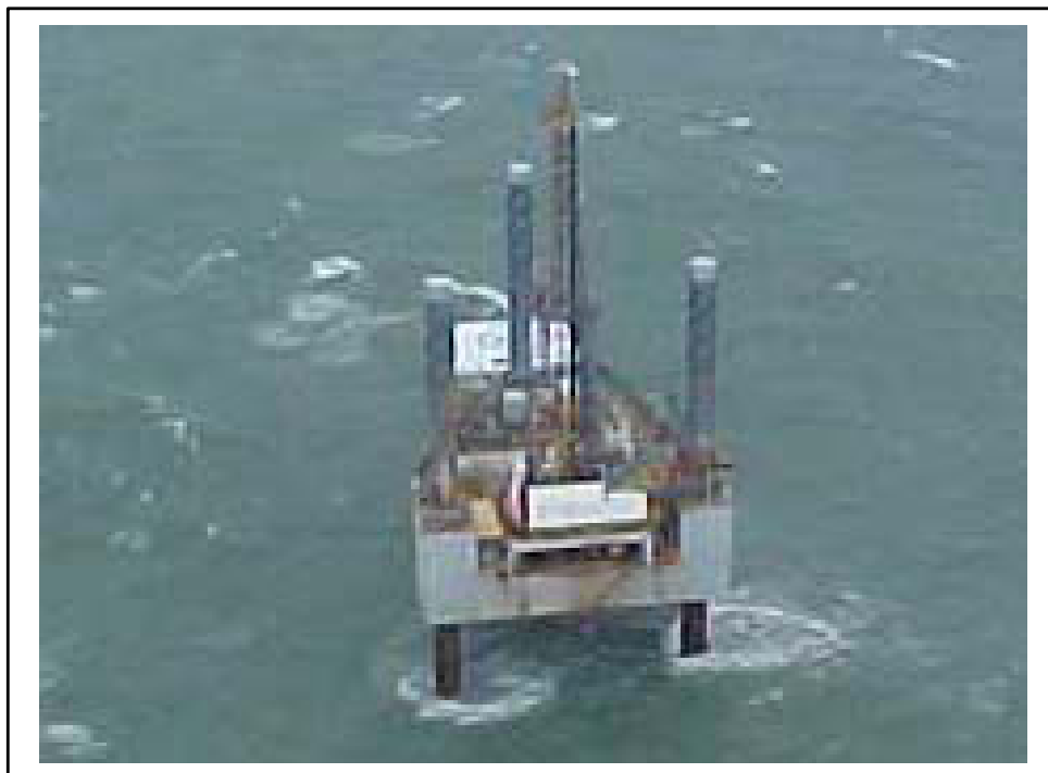
Figure 42: THE 200 Photo taken After the Storm (note effect of currents on the legs)
